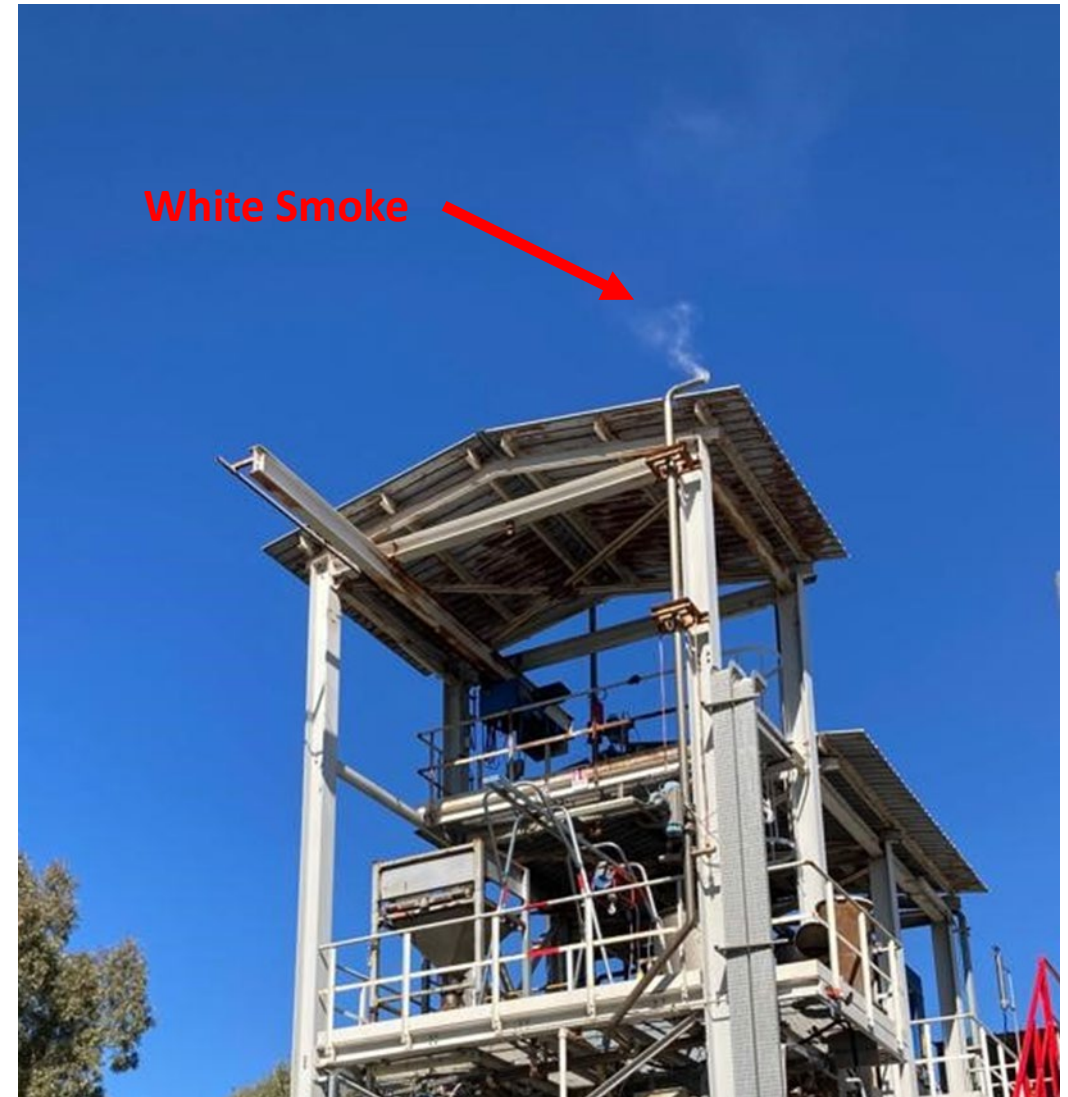
White Smoke From Vent Confirmed Ignition of the Gasifier
