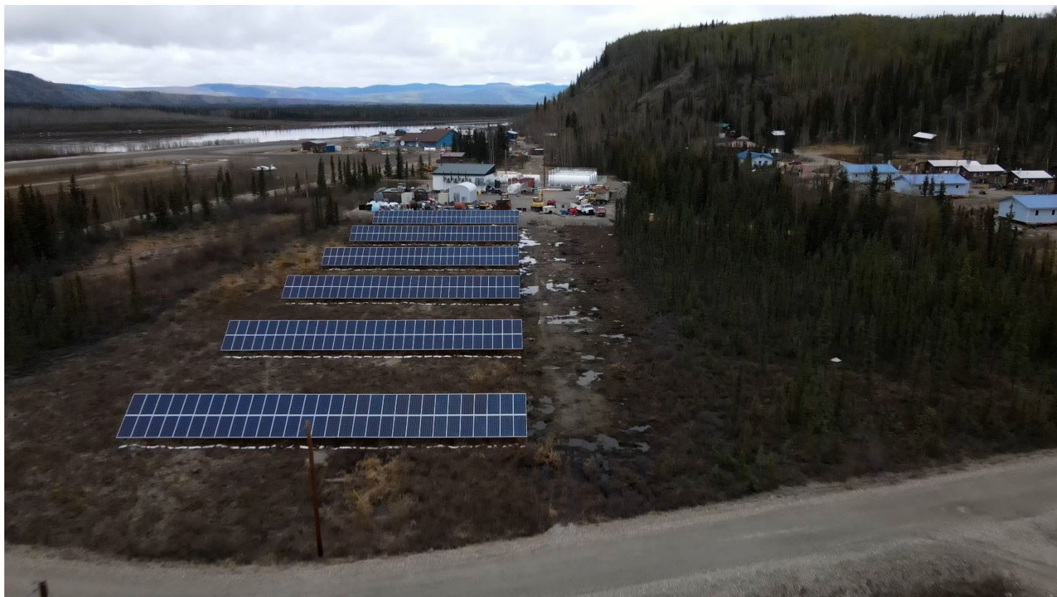
Figure 1. Aerial View of Solar Array with Battery Energy Storage System and Powerplant in the background
