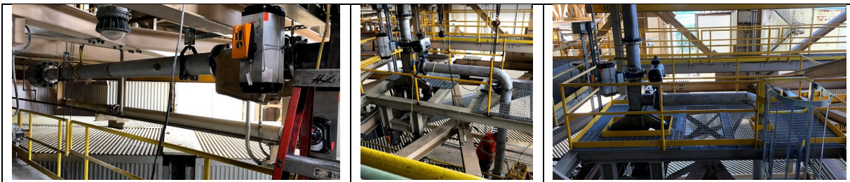
Exhibit 3.3.4. Air Inlet, Outlet Lines, Platform Grating, Handrail, and Ladder Installed.
