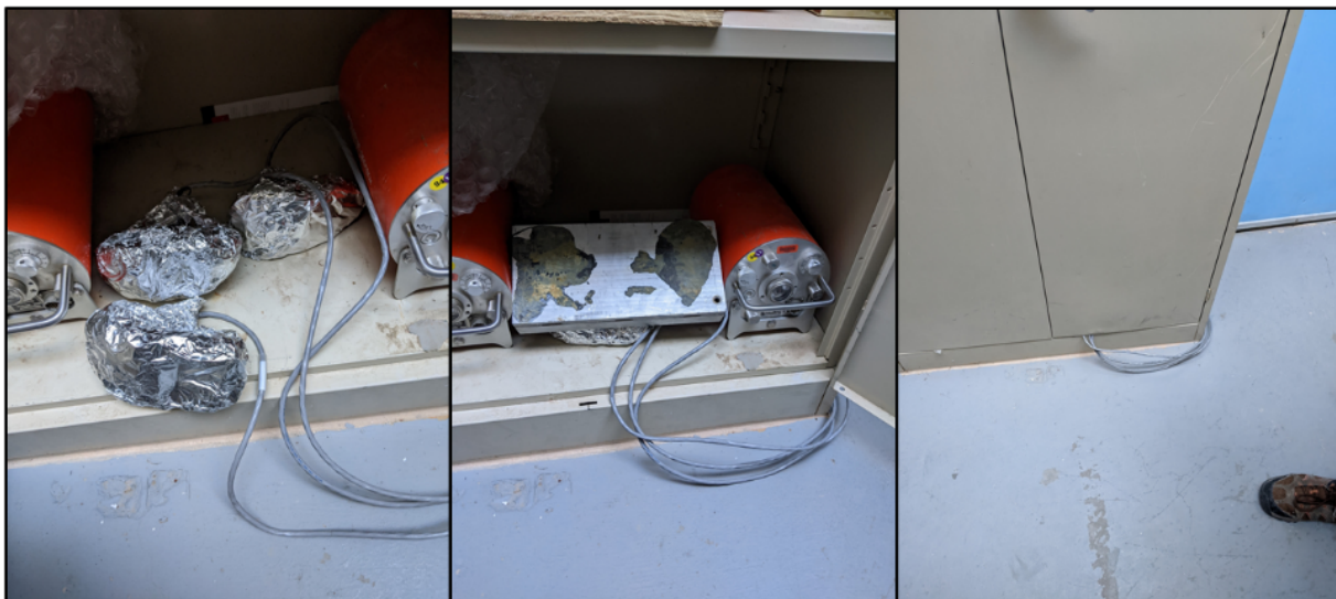
Figure 89 Timing Drift GNSS Antennas Shielded
