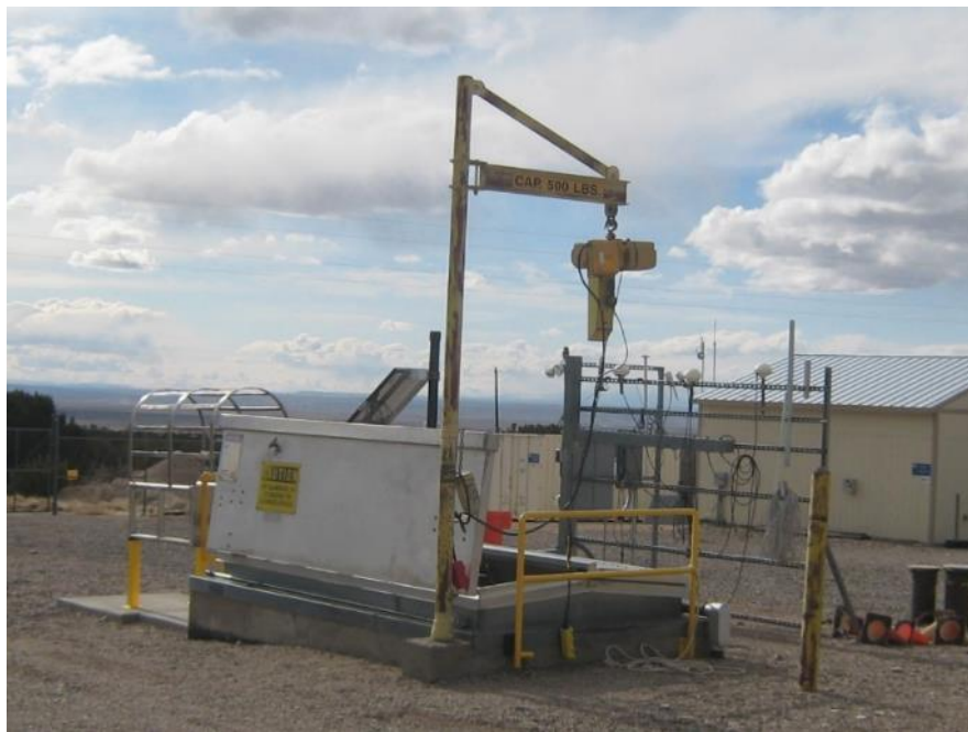
Figure 7 FACT Site Bunker
