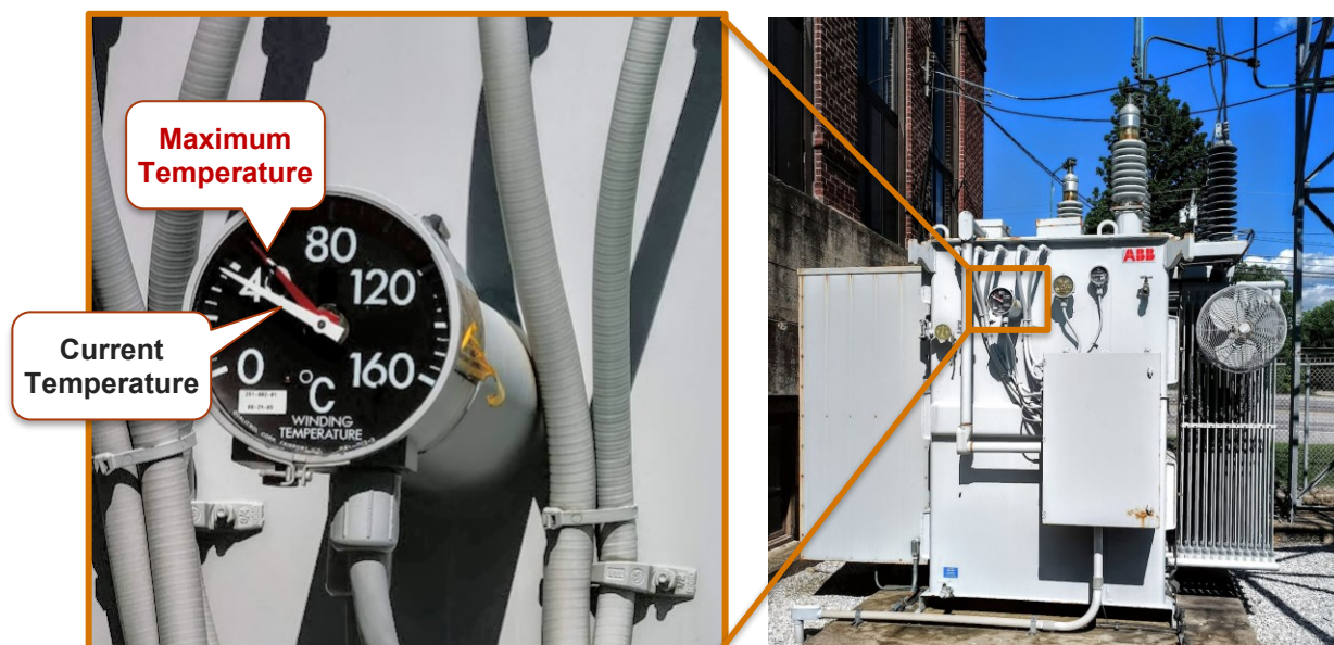
Figure 17: Closeup of a winding temperature gauge with the draghand needle indicating the highest temperature the transformer has reached since being reset.
