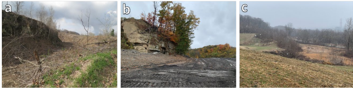
Figure 3-4 (a) Dewatered pit with exposed highwall (left) and mine spoil bank (right). (Photo by Cheng, April 2015). (b) Placement of sFGD (light gray in the left portion of the image) along the high wall and FA (dark gray in the right portion of the image) into the pit). (Photo by Martin, October 2022). (c) An example of completed reclamation is the application of mine spoil cap and revegetation with grasses (hay laid to prevent erosion) (Photo taken in October 2022).
