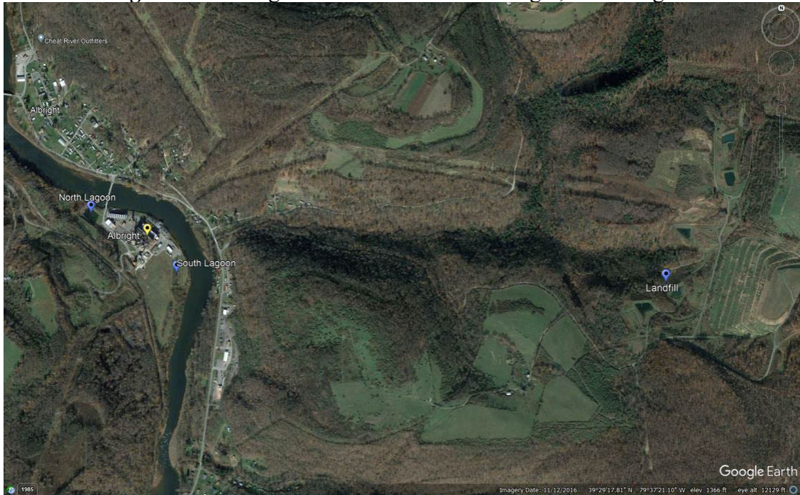
Figure 4-9. Albright Power Station near Albright, West Virginia
