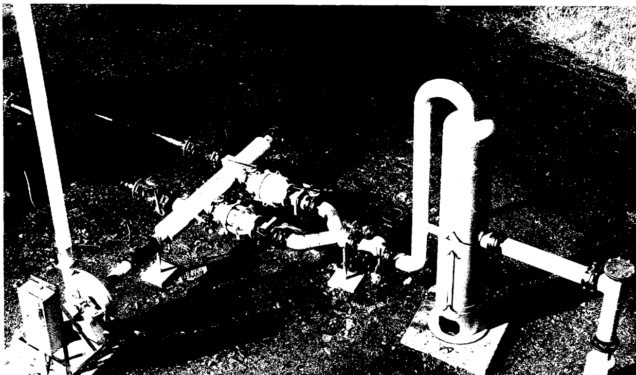
Figure 26 - Surface Facilities for a Medium Production Rate (1.2 MMcf/day) Gob Well
