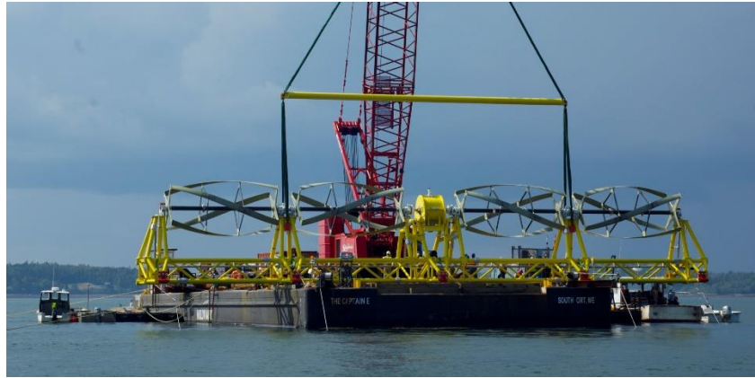
Figure 5: Cross-flow underwater turbine (Tethys Engineering n.d.)
