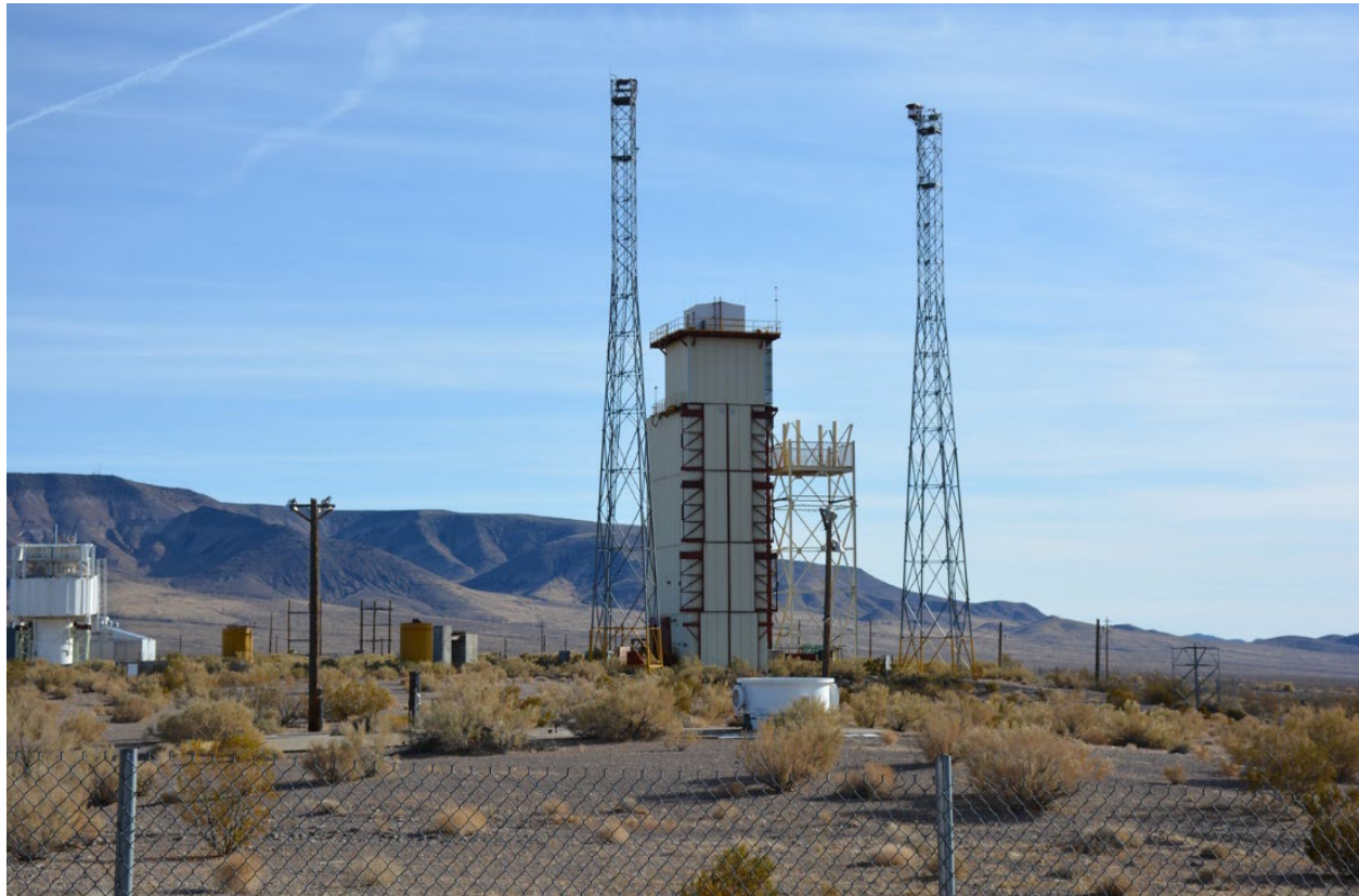
Figure 37. The MX Trial Launch Facility, facing south-southeast (Photo 2116_2024, DRI 2021). The enclosed tower held the missile launch canister. The two skeletal steel towers were for photography.
