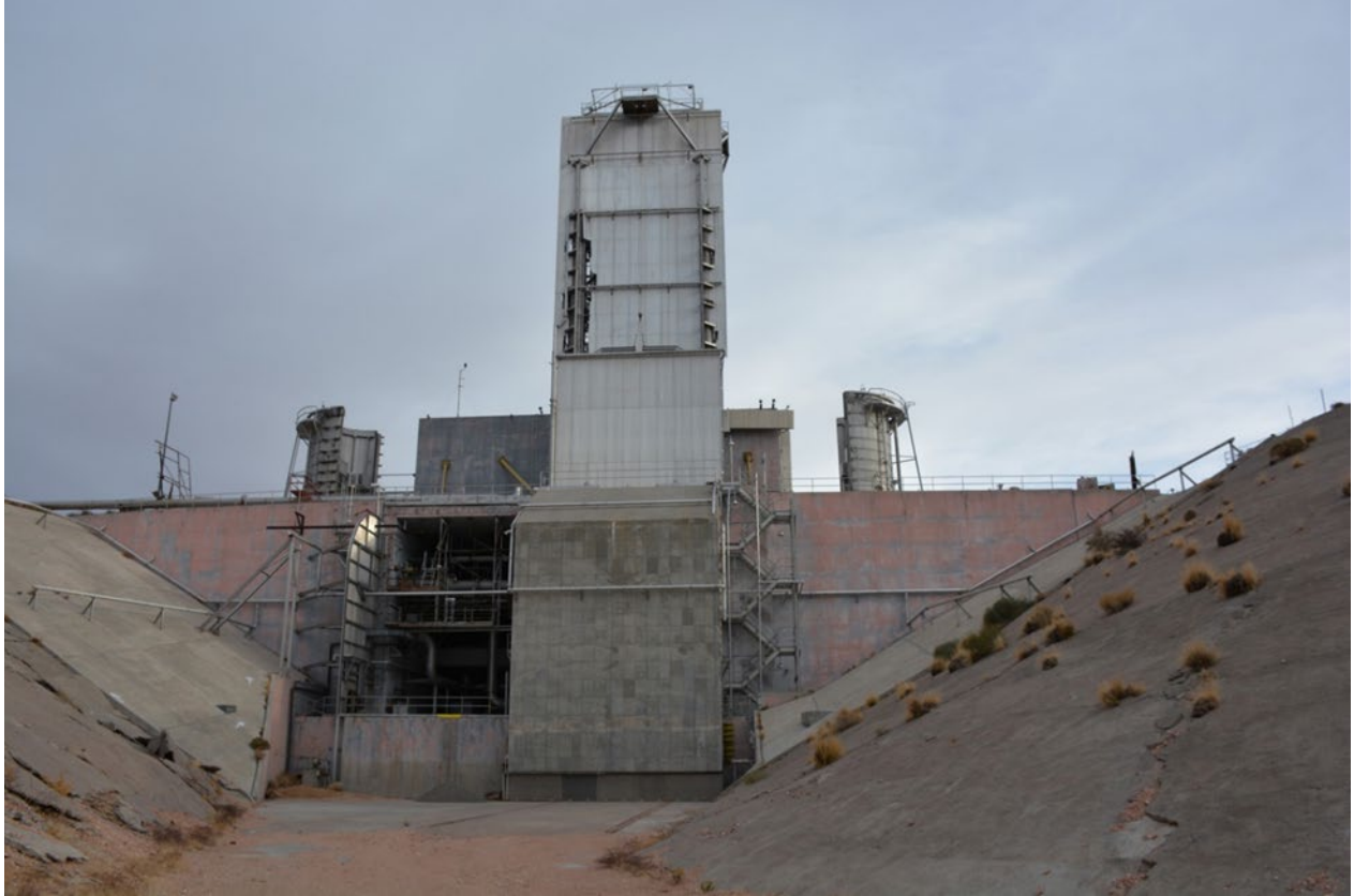
Figure 129. View of the north elevation of ETS-1 from the channel for the exhaust duct, facing southeast (Photo 2116_0848, DRI 2021). Pipes mounted on the walls of the channel and elsewhere are for water sprays.
