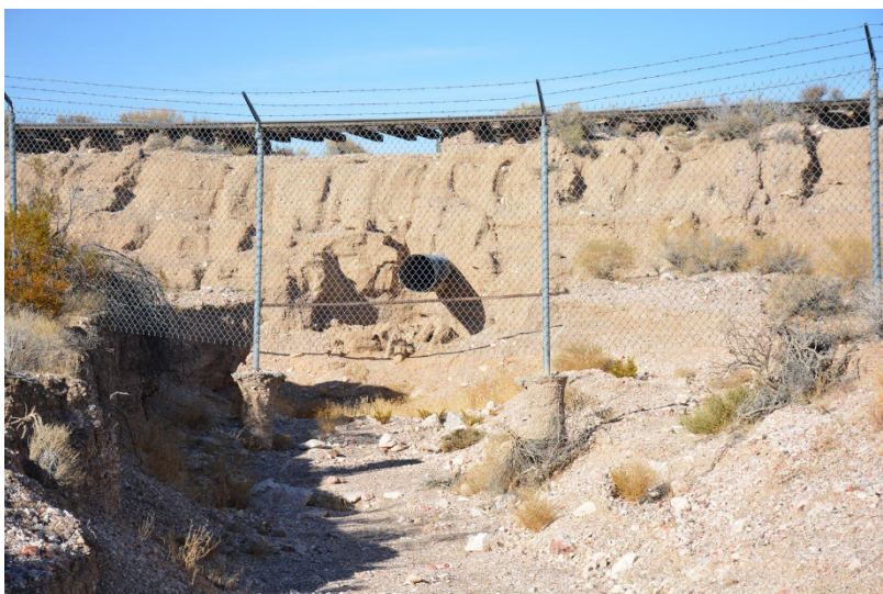
Figure 148. Washed out railroad subgrade at the RMSF, facing north (Photo 2116_2311, DRI 2021).
