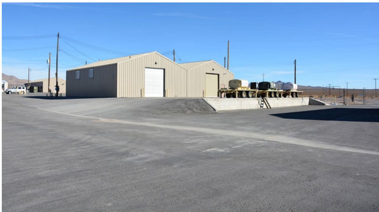
Figure 138. The rear of the warehouse area, facing northeast (Photo 2116_9284, DRI 2021). The downhill edge of the terrace for this warehouse was used as a loading dock. The framing of these steel buildings is original but exterior materials have all been replaced.
