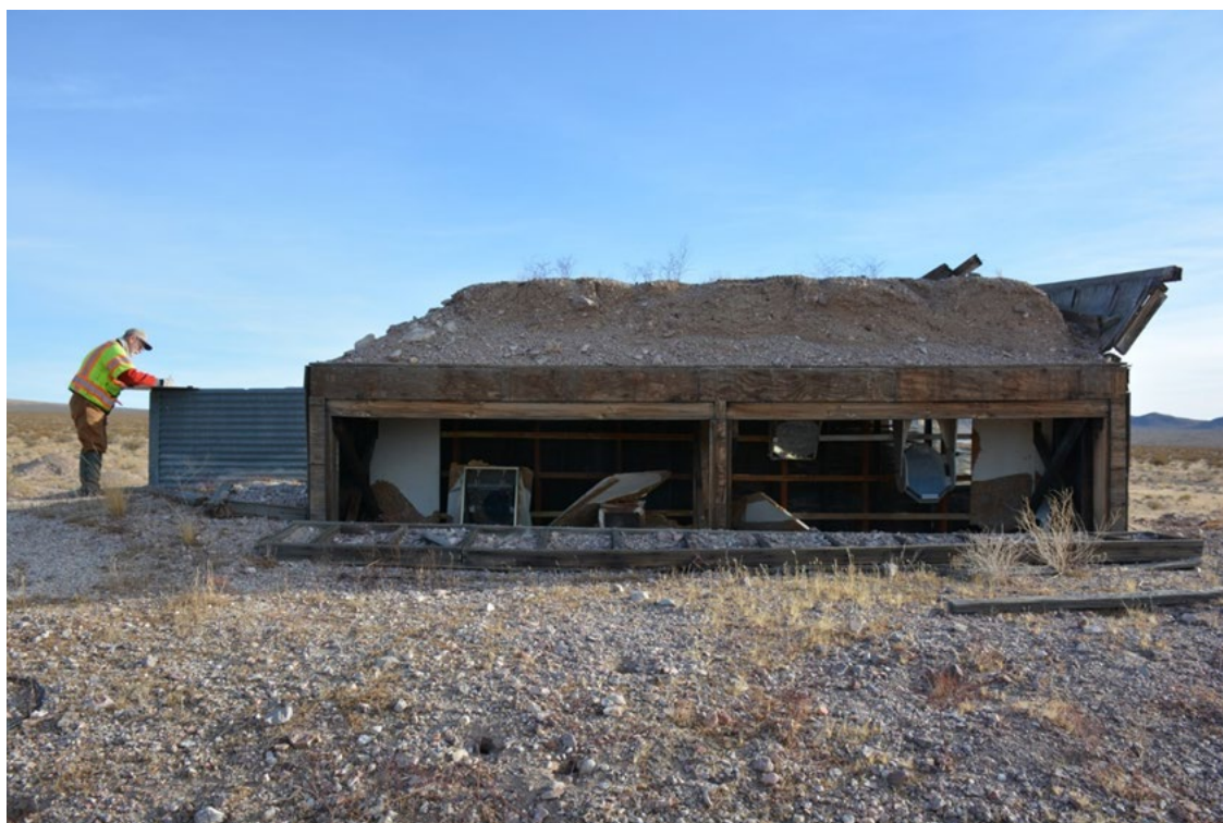
Figure 118. The Northeast Camera Station (B19023) at Test Cell A, facing north-northeast (Photo 2116_1716, DRI 2021). Periscopes are still present in the shelter. The worker is at the access shaft. Note earthen radiation shielding built into the roof.
