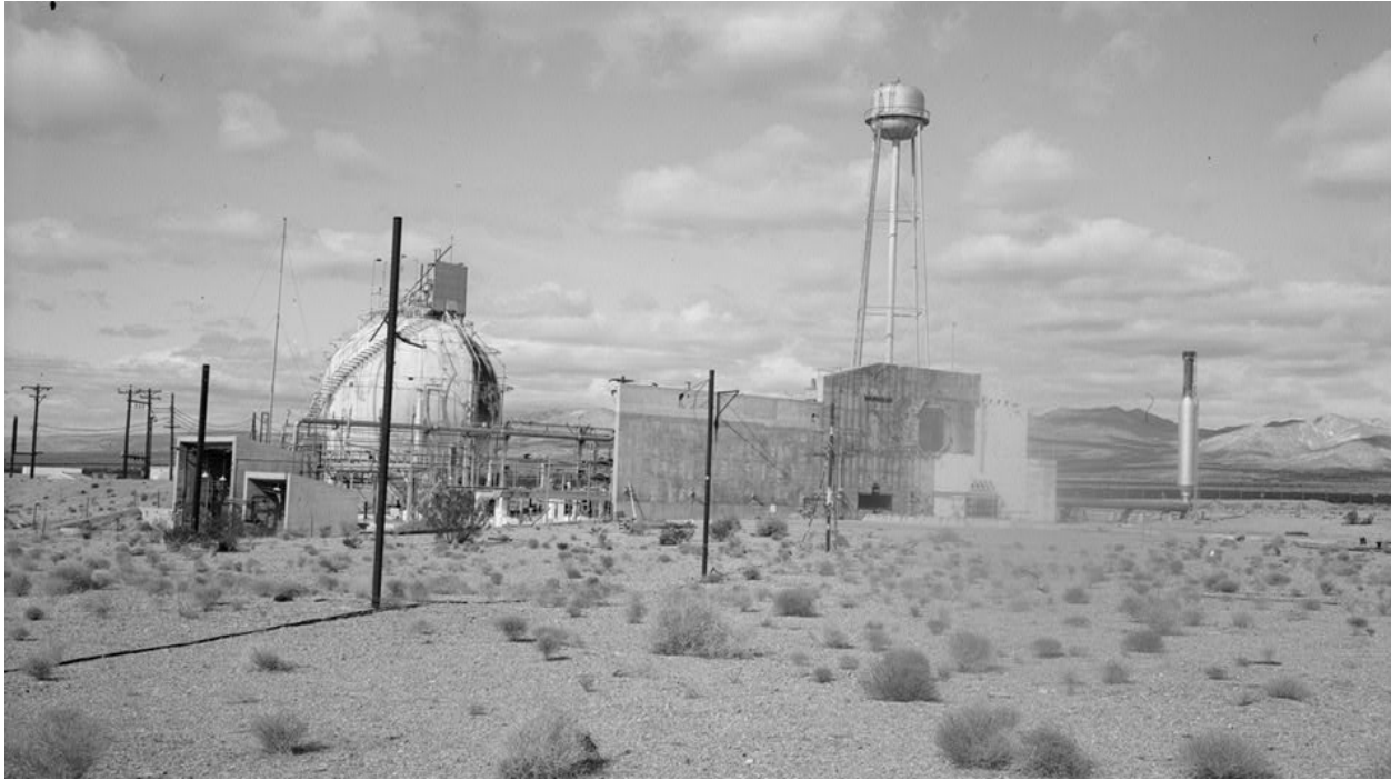
Figure 33. The Test Cell A Building before demolition, facing northwest (Beck et al. 2000, Photo 1). The shorter structure at left is the tunnel entrance. The hydrogen flare stack is at right.
