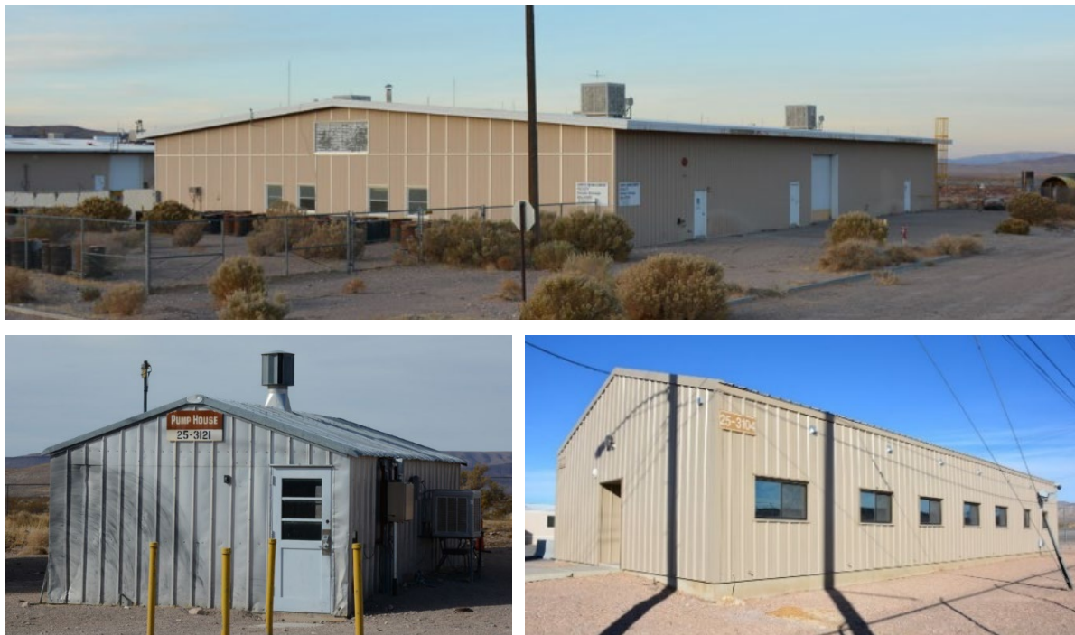
Figure 21. Examples of prefabricated buildings at the NRDS.
