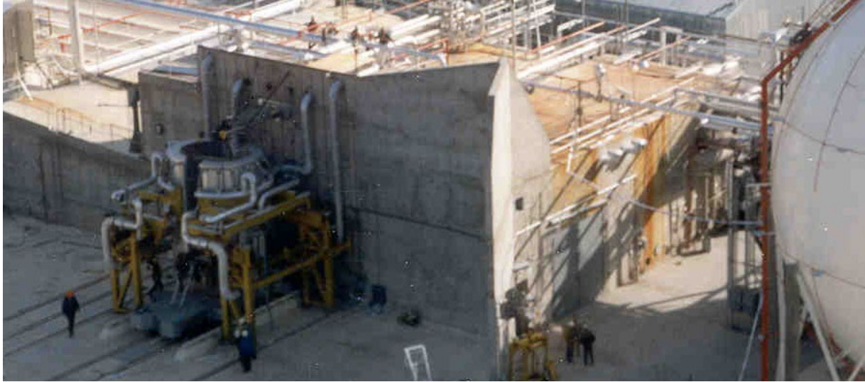
Figure 69. The protective concrete shield wall at Test Cell C is prominent in this view taken while preparing for a test (photo credit RSL c. 1997). The shield and the Test Cell Building behind it have been demolished. A portable clamshell radiation barrier surrounds the reactor in this image.
