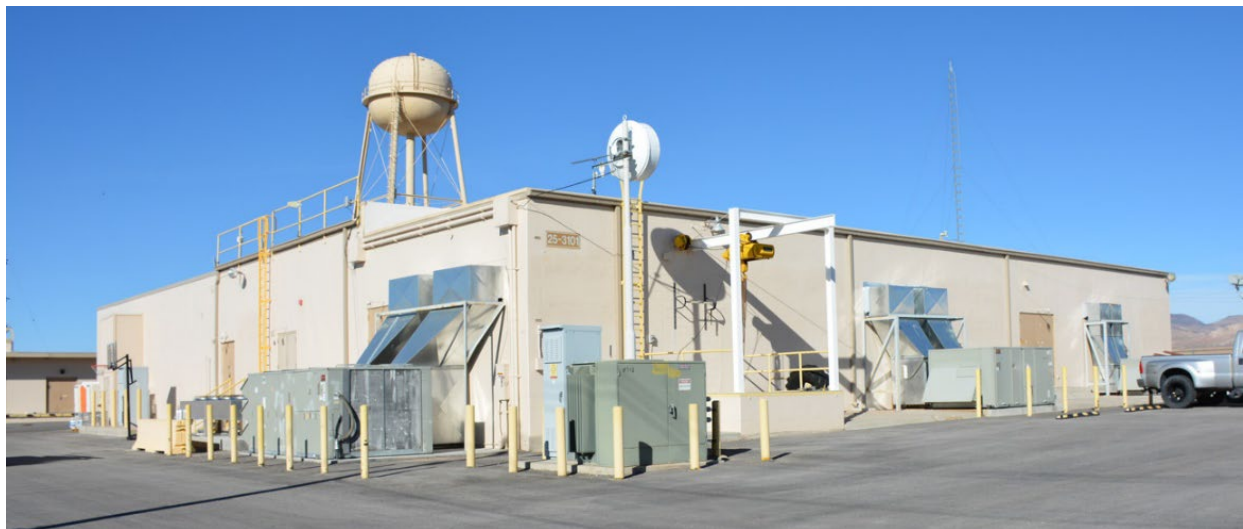
Figure 32. The RCP Control Building 25-3101 (B18993), facing northwest (Photo 2116_9300, DRI 2021). In the foreground extending over the roof is the overhead crane for moving equipment into and out of the basement.
