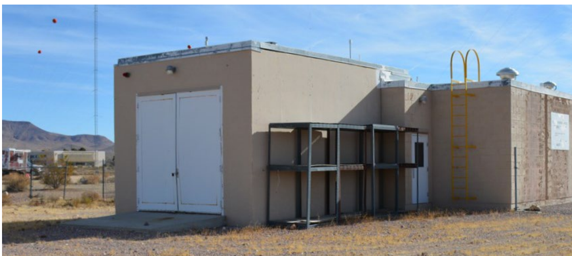
Figure 44. The Radiographic Bay at Building 25-4919 (B19020) has formed concrete walls up to 1 foot and 8 inches thick, image facing southeast (Photo 2116_1148, DRI 2021).
