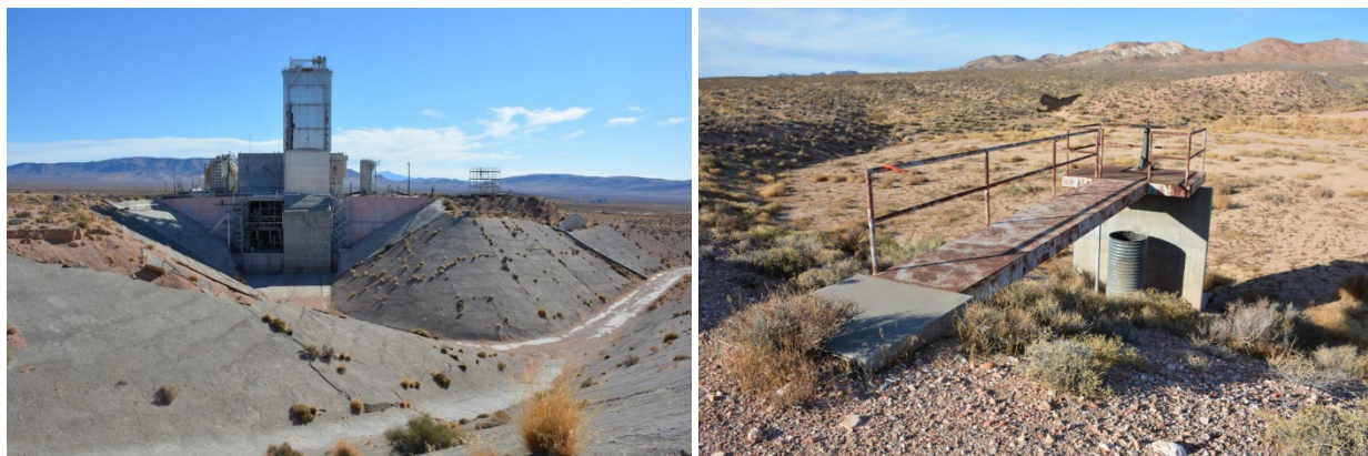
Figure 62. Deluge and water-cooling system at Engine Test Stand 1. Main drainage channel (Photo 2116_0232 [left]); containment reservoir (2116_0336 [right], both DRI 2021).
