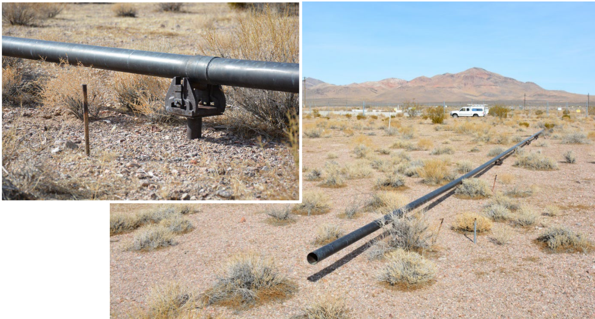
Figure 89. Cryogenic pipeline at Test Cell A (Photo 2116_1910, DRI 2021) with detail of roller mount for expansion and contraction (Photo 2116_1904, DRI 2021).
