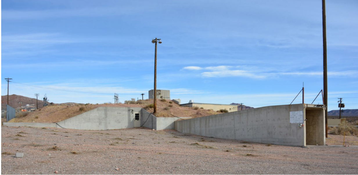
Figure 84. The Local Control Room in Building 25-3310 at Engine Test Stand 1 is underground for radiation and blast resistance (Photo 2116_0494, DRI 2021).
