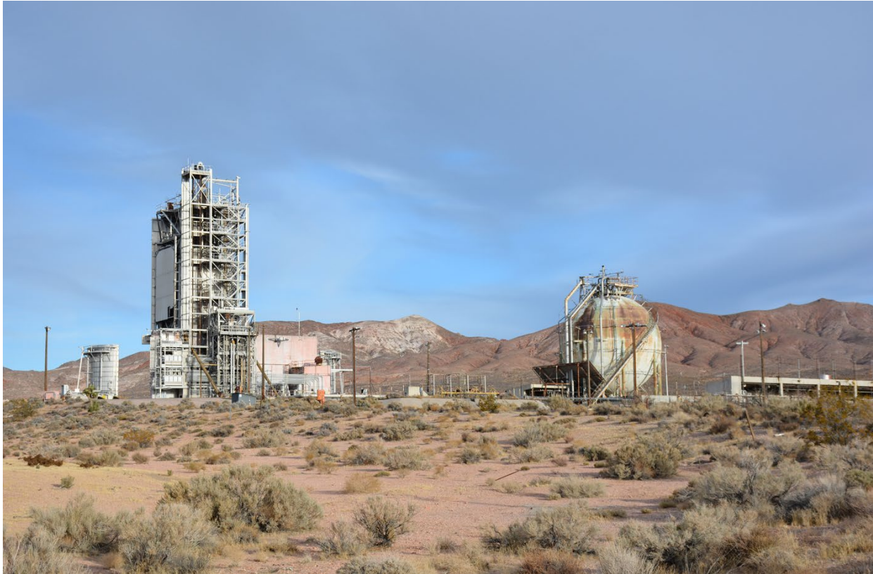
Figure 35. Engine Test Stand 1 and a portion of its Tank Farm, facing north-northwest (Photo 2116_9952, DRI 2021). The concrete radiation barrier wall is the pink part of the structure, mostly hidden behind the stairway and piping.
