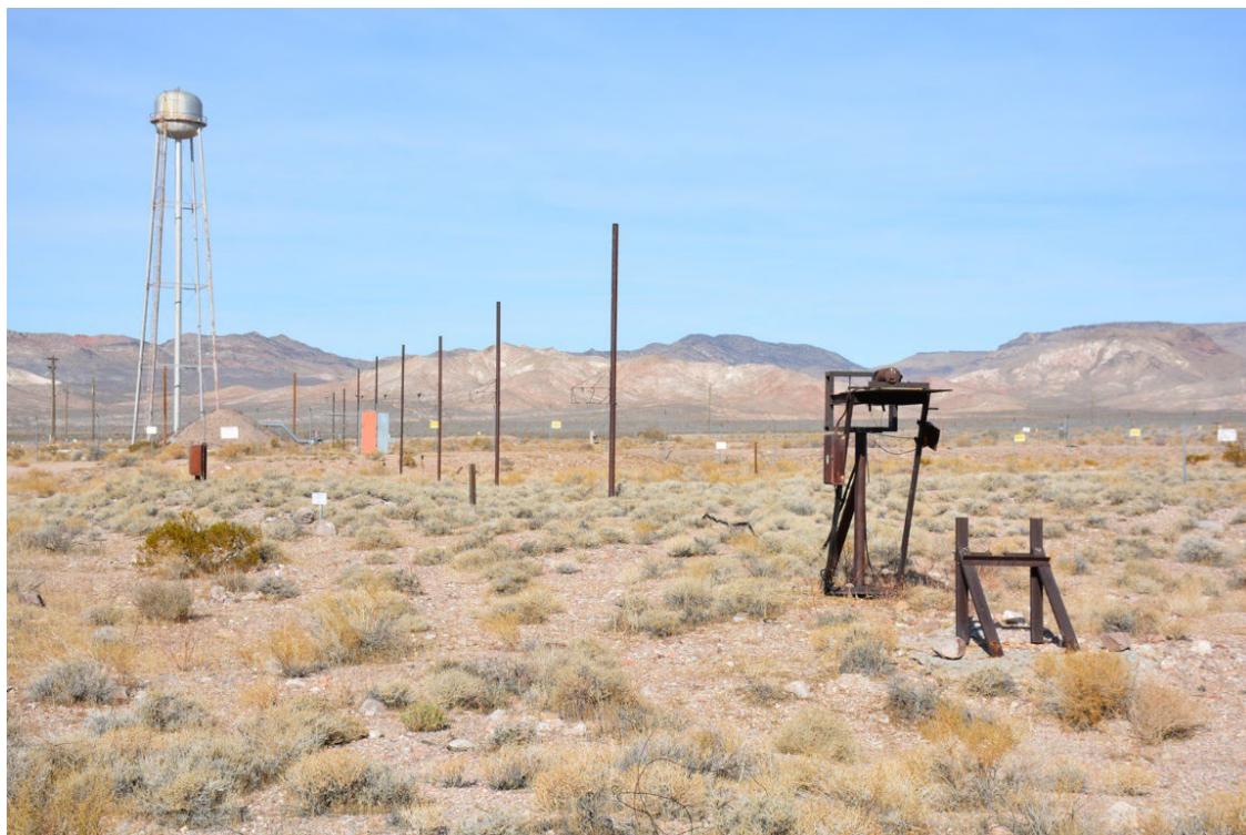
Figure 117. View northwest of the tramway showing upright steel pipes and a steel brace set in concrete at the southeast terminus (Photo 2116_1864, DRI 2021).
