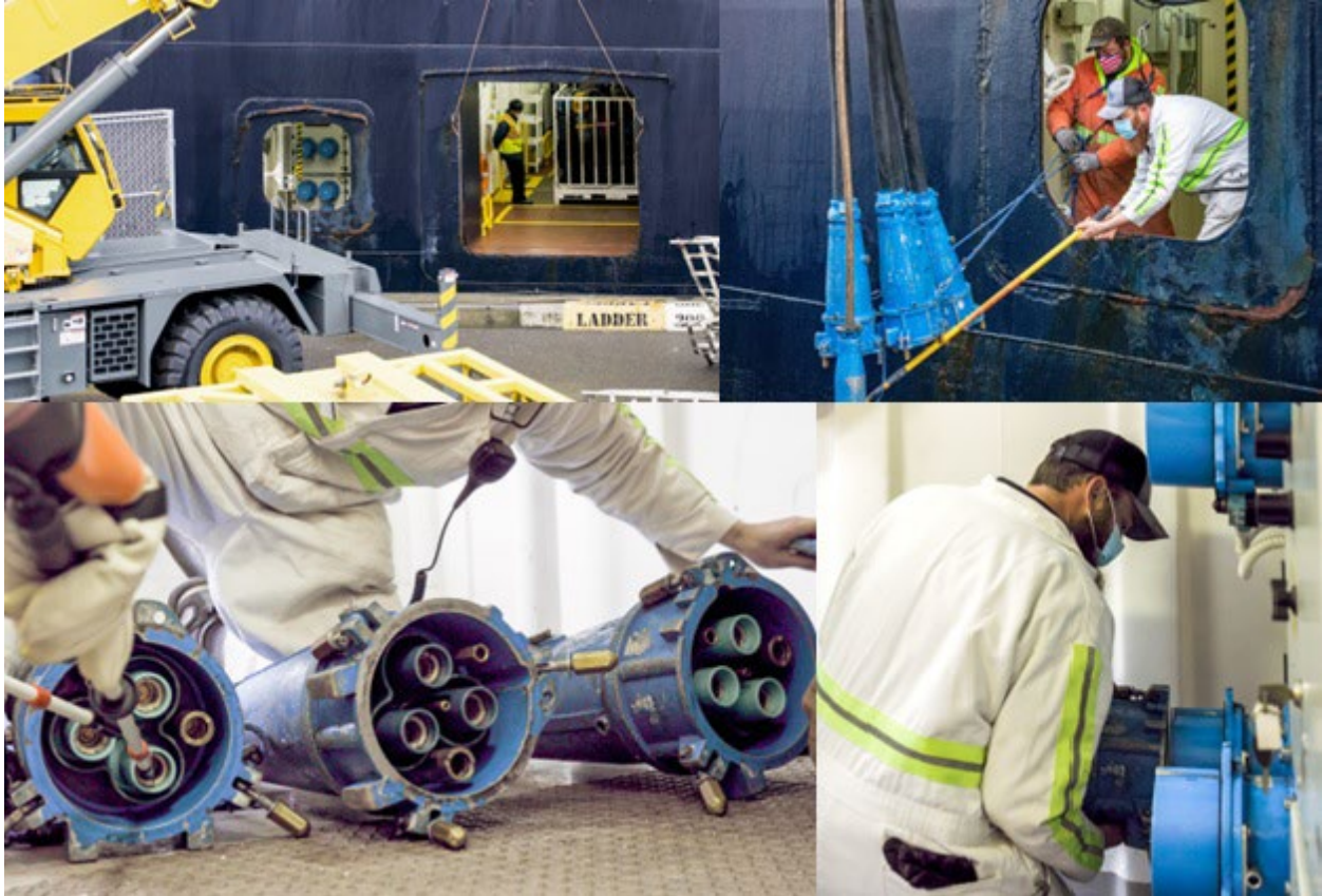
Figure 5. Compilation of images taken while plugging in a cruise vessel at the Port of Seattle. Photo Credit: Port of Seattle.
