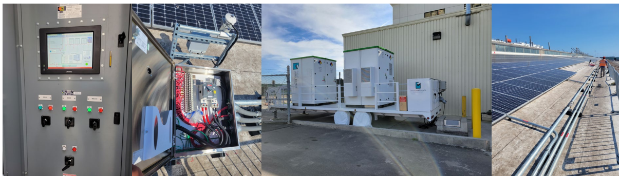
Figure 8. Left to right (1) main incoming board for the microgrid, (2) wiring for solar PV panel array, (3) microgrid-extending mobile BESS, and (4) 306 kW DC solar PV array on warehouse roof. Photo Credit: Port of Long Beach.
