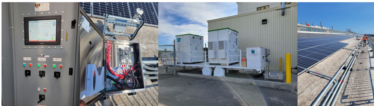
Figure 24. Left to right (1) main incoming board for the microgrid, (2) wiring for solar PV panel array, (3) microgrid-extending mobile BESS, and (4) 306 kW DC solar PV array on warehouse roof. Photo Credit: Port of Long Beach.
