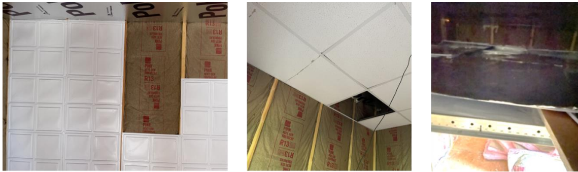
Figure 12. Installation trials of PCM wall panel application - PCM 22°C (right), and PCM suspended ceiling installation - PCM 22°C – bottom view, conventional appearance (center), and top view (right).
