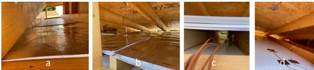
Figure 13. Installation trials of two PCM attic systems; (a) top of the ceiling installation - PCM 29°C, (b) attic cavity installation - PCM 22°C, (c) instrumentation of attic cavity below PCM, (d) instrumentation of comparative, conventional, baseline attic.
