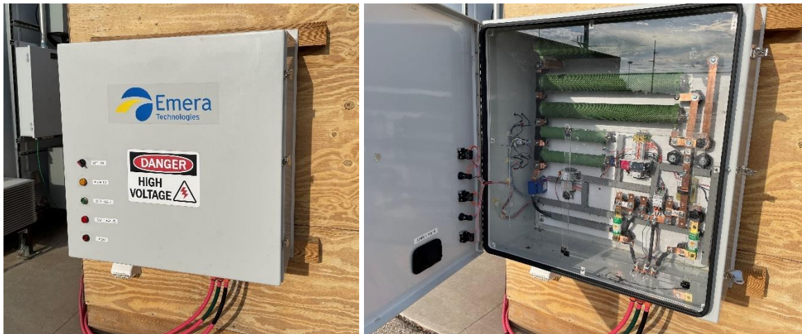
Figure 153. Fault emulator hardware installed onto microgrid distribution bus at the DETL.
