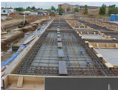
Tilt-Up (site prefabricated)
