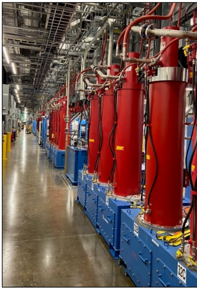
Figure 2: RF systems to power the new cryomodules.
