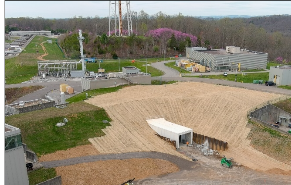
Figure 5: RTBT tunnel stub for connection to the STS.
