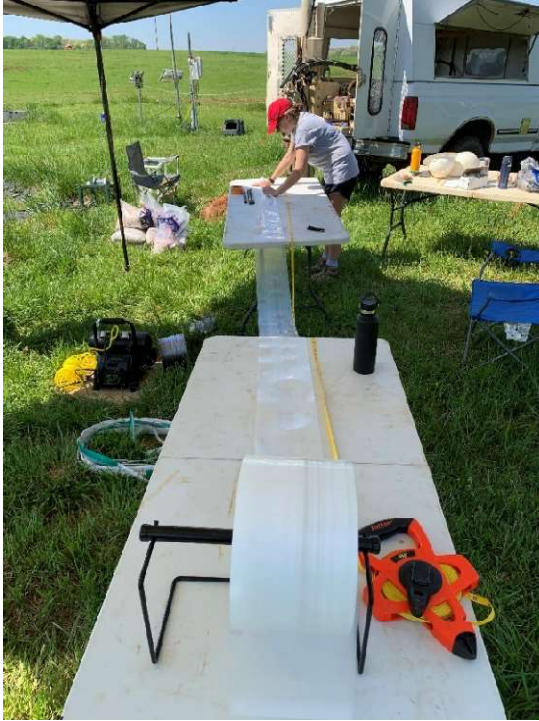
Figure 2.7: Polyethylene sleeve being prepared for installation in the borehole. a: Tubing meaning measured. b: Tubing being folded.
