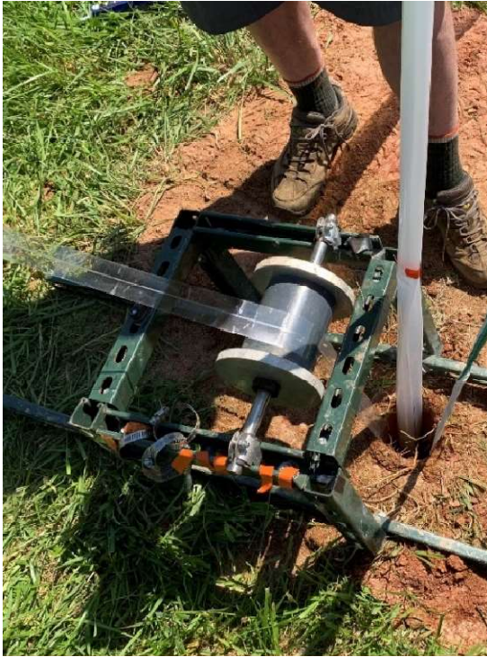
Figure 2.8: Installation of the polyethylene tubing in the borehole. a.) Strain ribbon (transparent) passing over a roller at the top of the borehole. Folded polyethylene sleeve is the white band at the top of the image; b.) Close up of the borehole with the transparent strain ribbon and the folded polyethylene sleeve.
