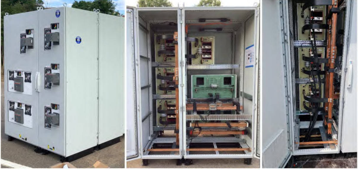
Figure 21: (Left) Corner view of the switchboard; the two larger line-side breakers on the bottom left. (Middle) Rear view, with doors opened. (Right) Load side cable connections shown at NYPA Pilot in Marcy, NY.
