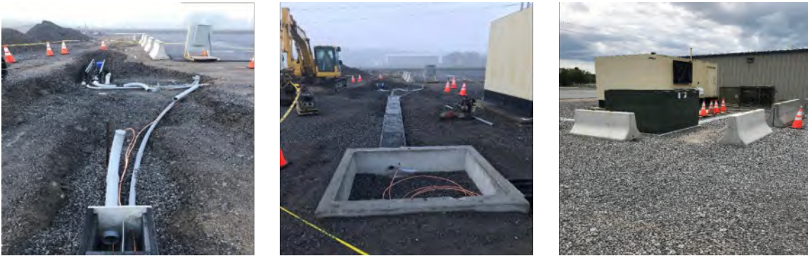
Figure 35: Preparatory work completed prior to the delivery of the shipping container at the NYPA Clark Energy Center site. Left: conduit placement; Middle: placement of Trenwa trenches and concrete for the placement of switchgear. Right: completed installation of the MV switchgear.
