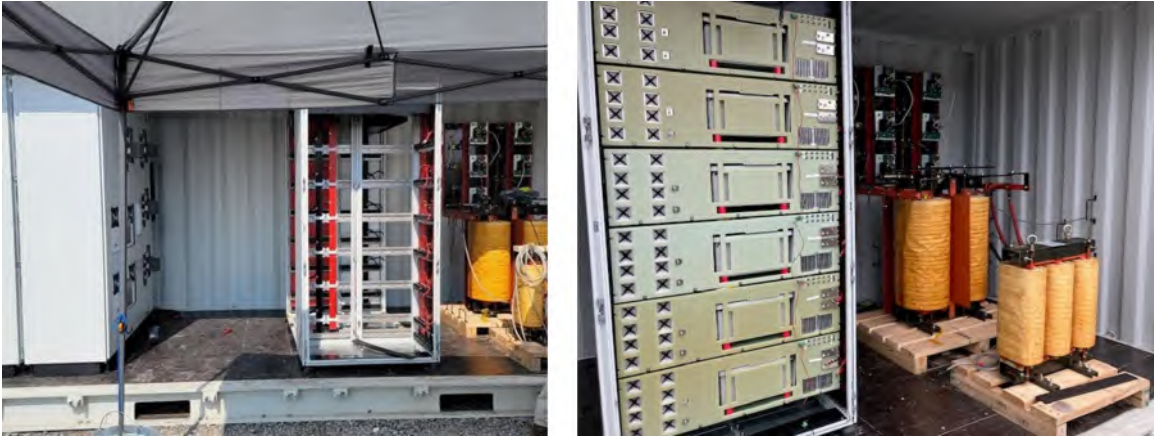
Figure 38: Shipping container during various phases of the commissioning process. Left: Shipping container prior to the placement of XFC modules inside the Module rack. Right: Shipping container detail, with SST modules in place.
