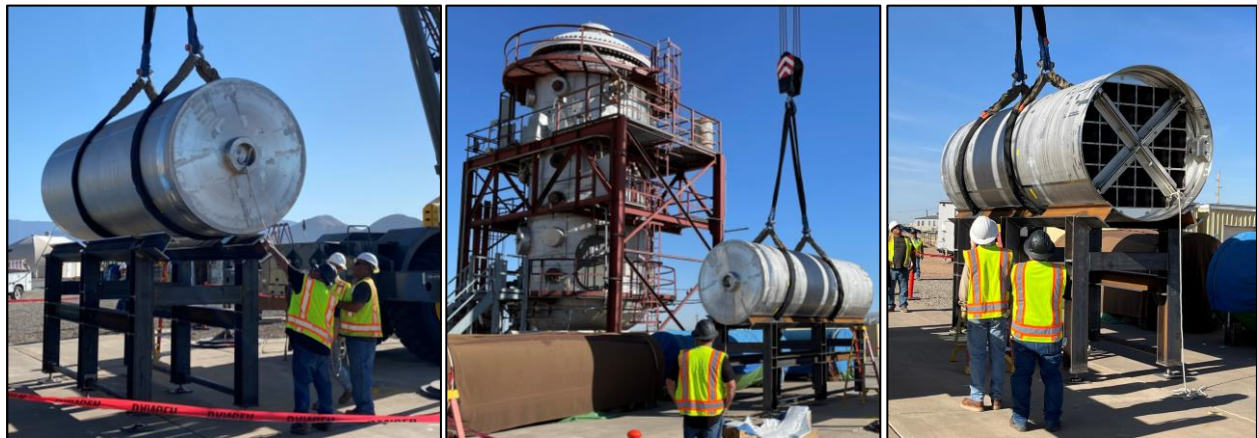
Figure 2.32 Placement of 32PTH2 dry shielded canister onto standoff.
