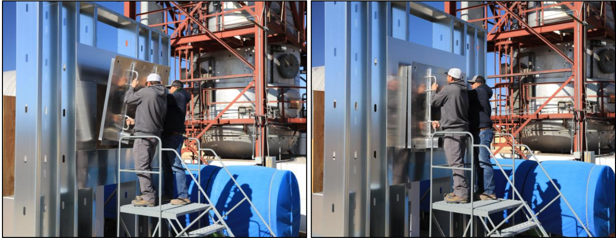
Figure 2.40 Dry fit of the rear access hatch cover.
