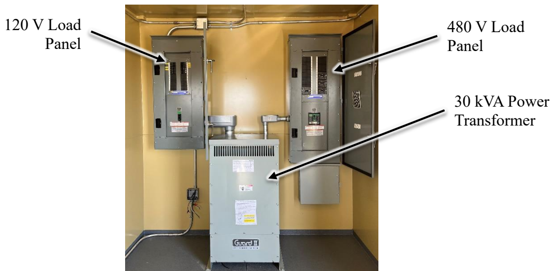
Figure 4.3 Rear wall of the power and instrumentation skid showing the 120 V load panel for data acquisition and accessory equipment power (left), 30 kVA power transformer (center), and 480 V load panel for heater assembly power (right).
