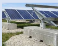
Piles in concrete
