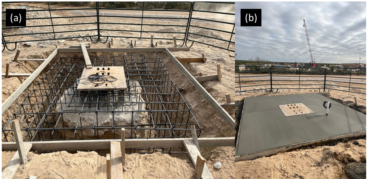
Figure 2.6 (a) Rebar cage installed during the repair of SOV2, and (b) SOV2 after placement of concrete.
