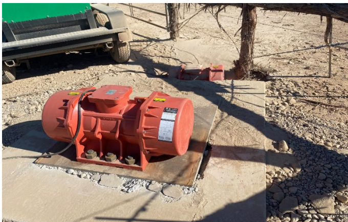
Figure 2.4 Degradation of the SOV2 foundation. Note that the small motor has sheared the hold-down bolts and is located beside the concrete pad. The above picture shows a large void under the steel plate and a significant degradation of the concrete around the plate.
