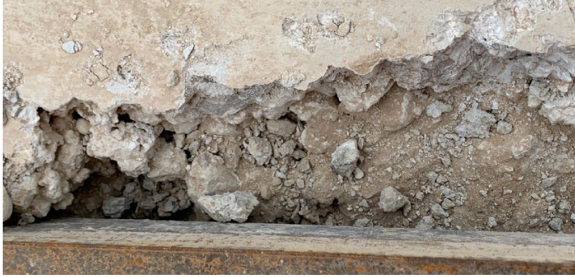
Figure 2.5 Close inspection of the SOV2 foundation revealed that the concrete had begun hydrating prior to placement, and large voids and vugs were observed.
