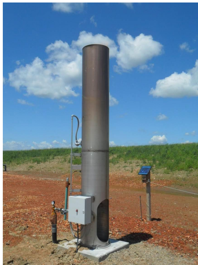
Figure 15. Example of enclosed combustor, from [71].
