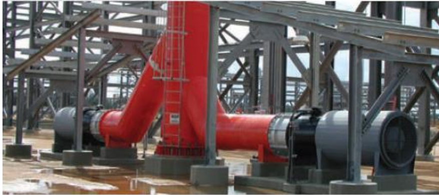
Figure 34. Air-assisted flare blowers, from [113].
