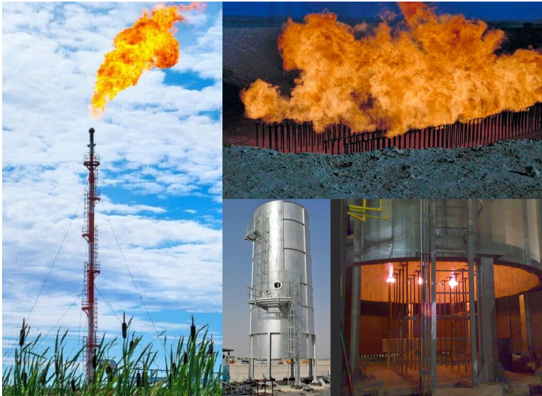
Figure 14. Flare types, elevated flare (left, from [69]), ground flare (upper right, from [70]), enclosed ground flare (bottom right, from [70]).
