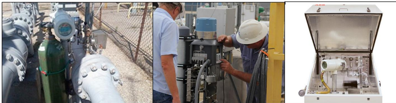
Figure 50. Examples of inline GCs for natural gas compositional analysis, from [159].
