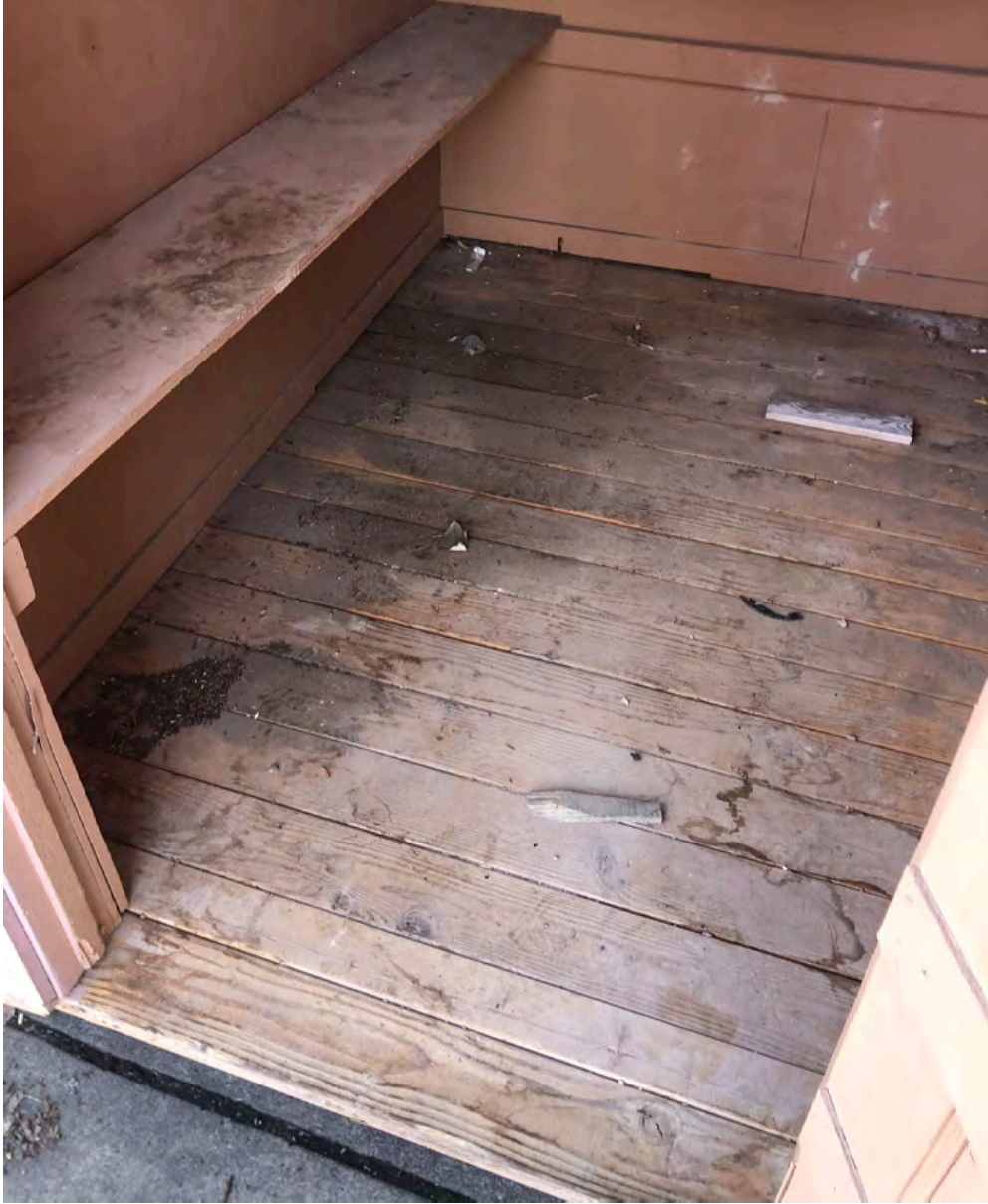
The interior 2" x 6" floor deck in TA-18-111.
