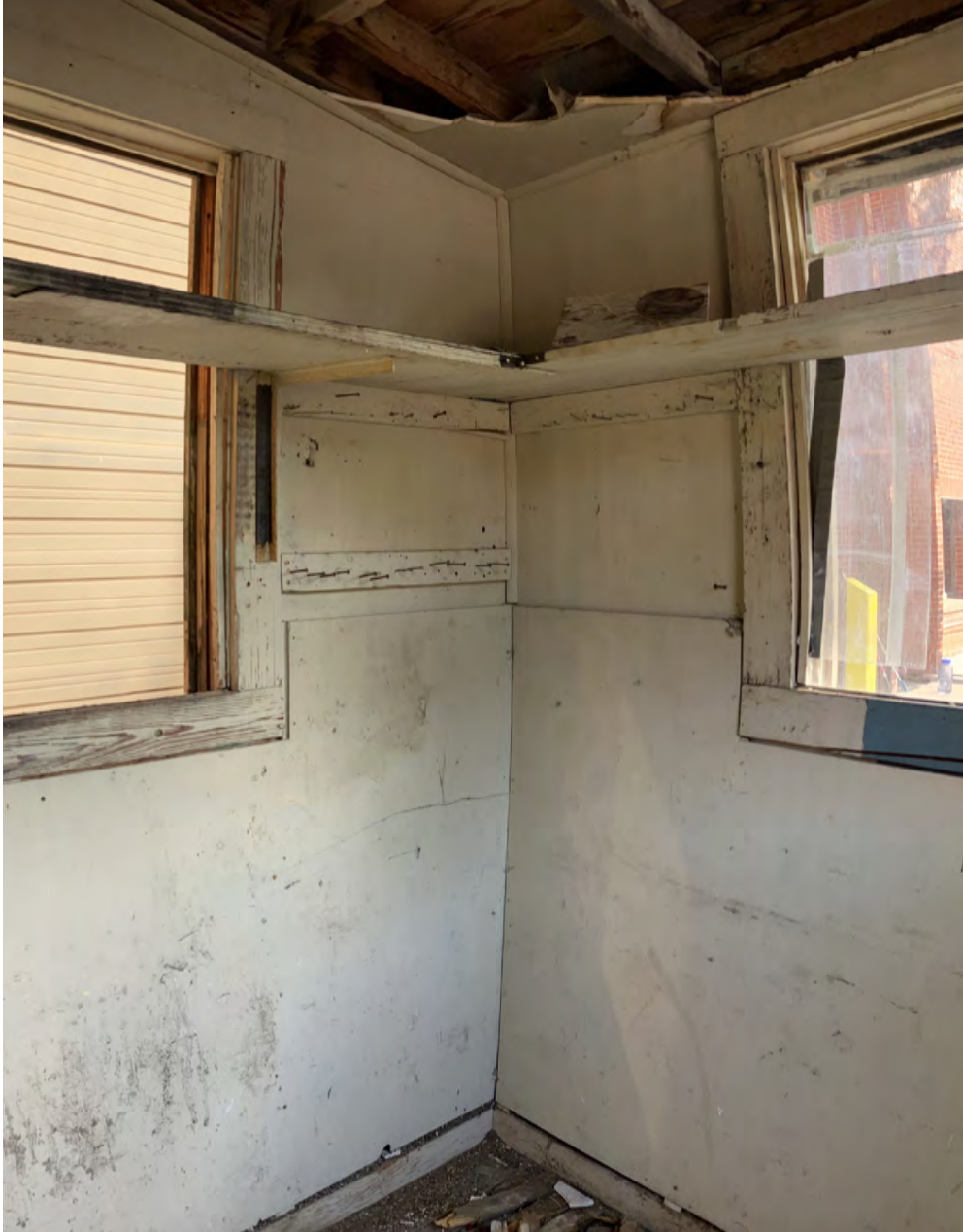
The interior of the back left corner.
