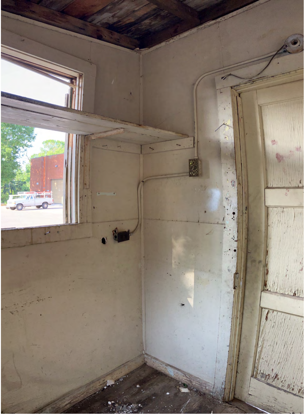
The interior of the front right corner.
