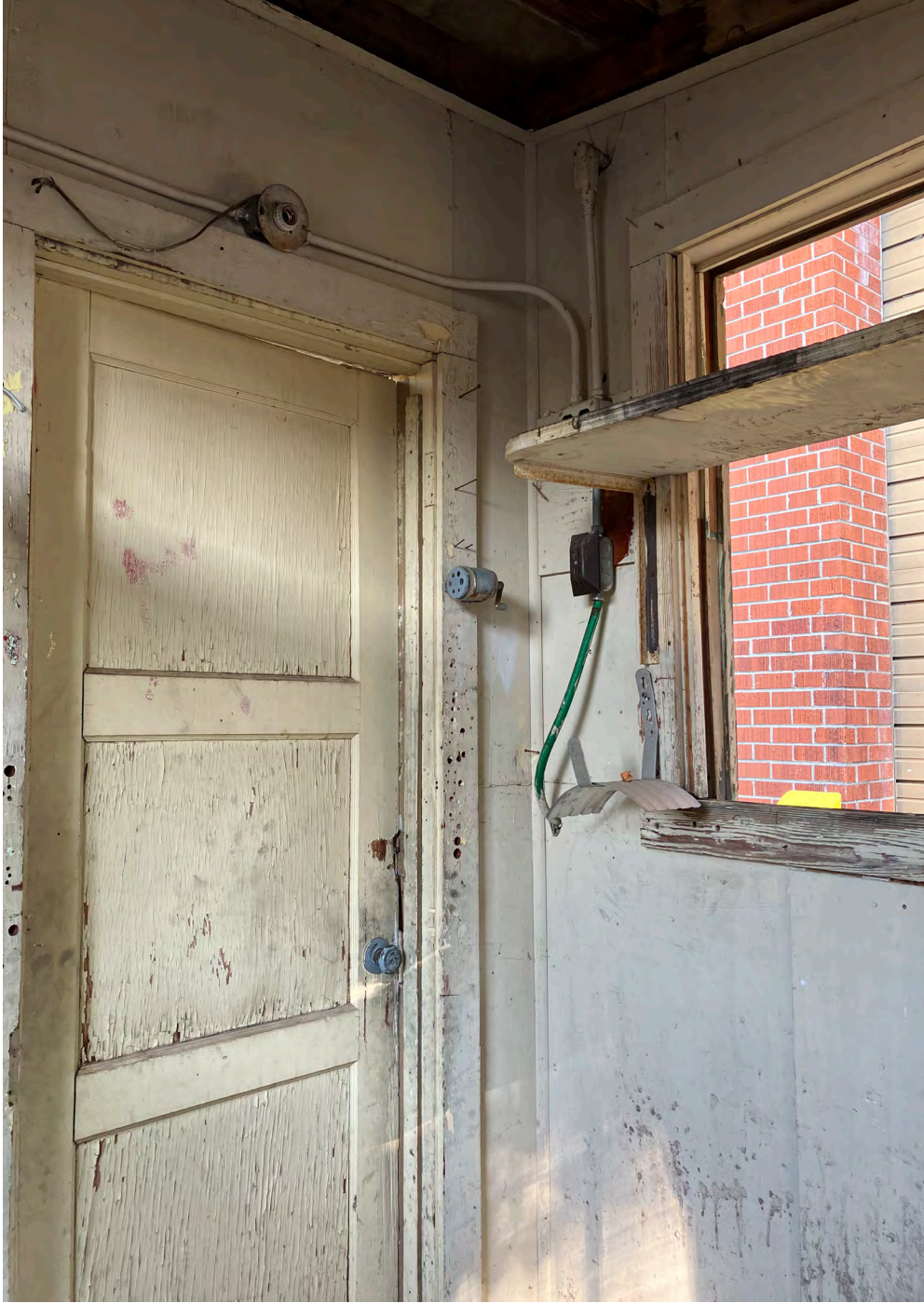
The interior of the front left corner.
