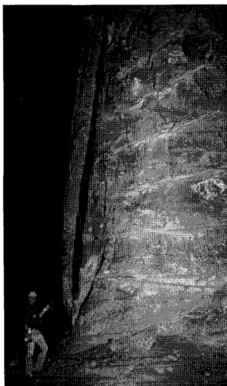
Figure 2. Photograph of a spalling pillar in the Markel Mine.
