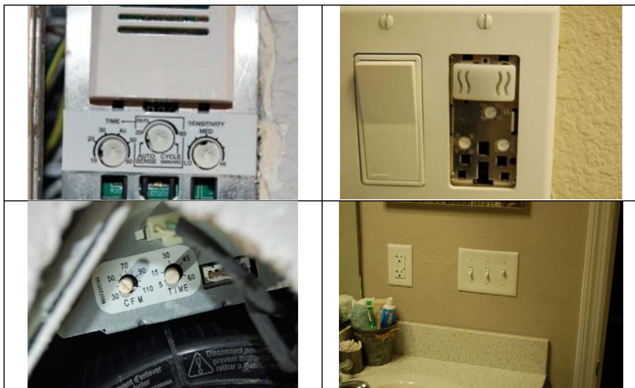
Figure 4. Examples of exhaust fan controls. Top – runtime and relative humidity controls located on switches. Bottom left – flow controls located on fan. Bottom right – wall switches that enable standard and boost operation.
