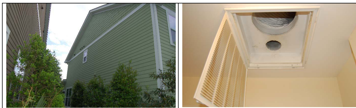
Figure 6. Left – CFIS outside air intakes high on wall are difficult to access for commissioning. Right – this return plenum ducting arrangement generates little flow through the 4-in. outside air duct.
