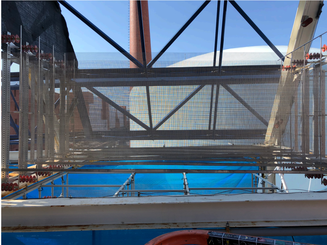
Figure 24: Infinite Cooling WaterPanel™ design installed at MIT NRL Site 2
