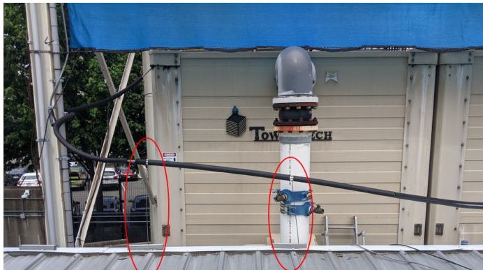
Figure 27: The reattached pipe for collected water with a steeper angle (set by choosing longer attachments circled in red) to prevent future clogging.
