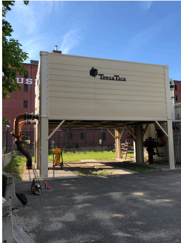
Figure 22: MIT NRL cooling towers – 25ft TowerTech cooling towers
