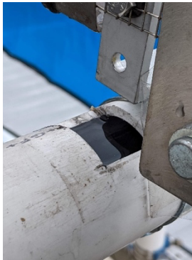
Figure 26: Overflowing pipe due to clog lower in the system
