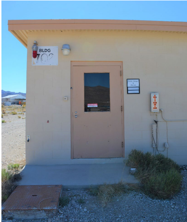
Figure 16. North elevation entry door, lighting, signage, and communications equipment, facing south (2360_0094, DRI 2023).
