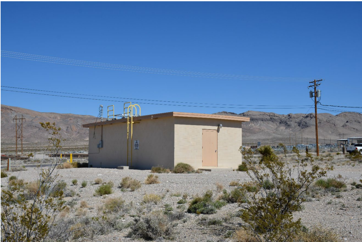
Figure 15. Building 23-702, south and west elevations, facing northeast (2360_0091, DRI 2023).
