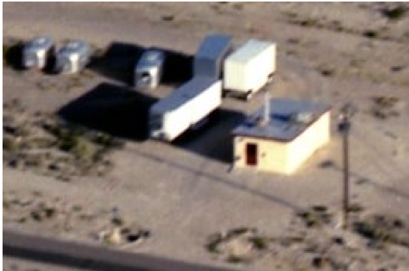
Figure 13. Aerial image showing Building 23-702 in 1991 (best copy available; modified from National Archives [1991], id 75491325).
