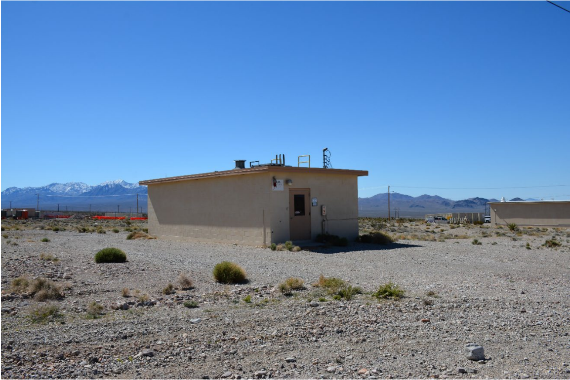
Figure 14. Building 23-702 north and east elevations, facing southwest (2360_0087, DRI 2023).
