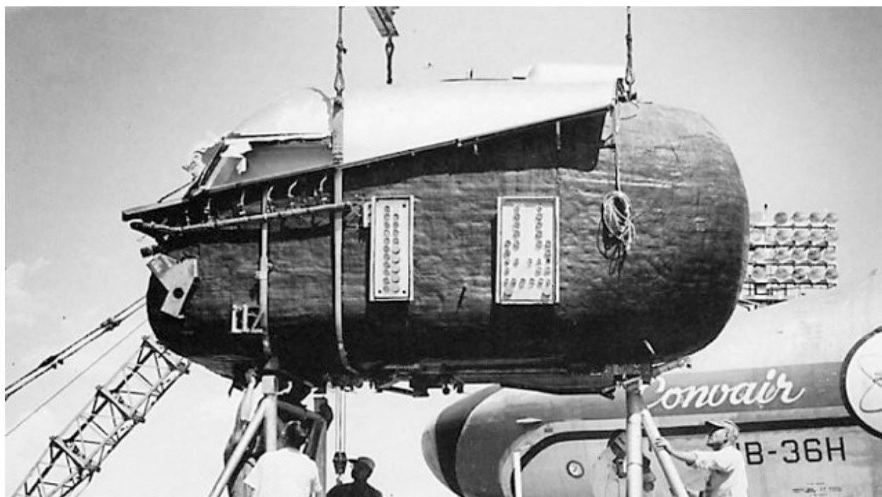
Figure 3. NB-36H Shielded Crew Compartment
