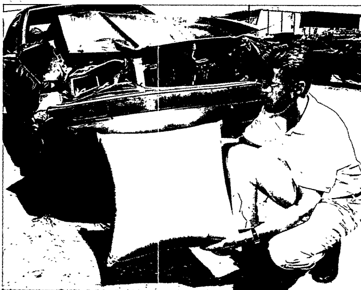
Sandia researcher Kenneth Gwinn displays a prototype of the compact, lighter airbag developed by Sandia and Precision Fabrics Group.
