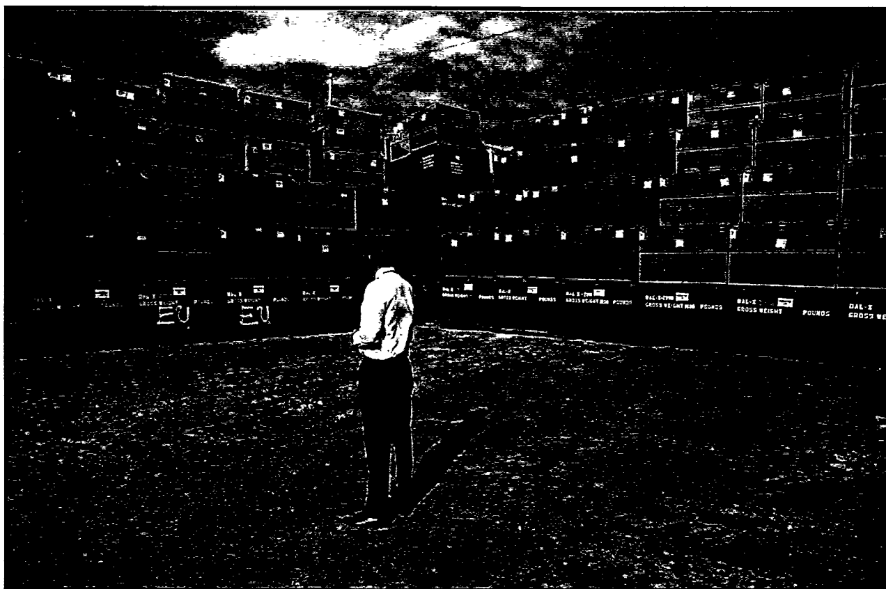
Boxes containing low-level radioactive waste lie in a shallow land burial trench at the Savannah River Site. New methods for disposal of low-level waste are being developed by the Department. Savannah River Site, South Carolina. January 7, 1994.
