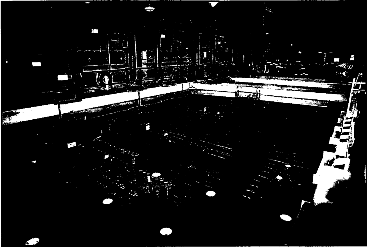
Pool for the storage of spent fuel. This pool is 28 feet deep; 7 feet of water cover the top of the highly radioactive spent-fuel elements. Water cools the fuel and also acts as radiation shielding. Receiving Basin for Offsite Fuel, Savannah River Site, South Carolina. January 7, 1994.
