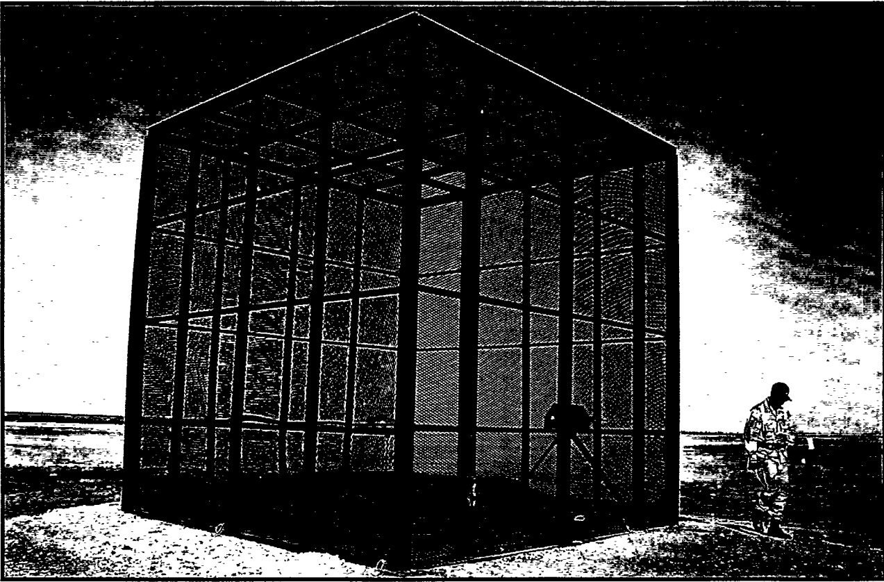
A burn cage is used at the Pantex site to dispose of items associated with the shipping and handling of high explosives used to make nuclear warheads. Wooden and cardboard crates and other materials contaminated with high explosives are burned inside the cage. Burning ground, Pantex Plant, Texas. November 18, 1993.
