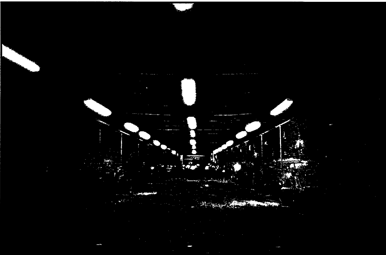
This underground waste-disposal room, excavated in 1986, was the first of 56 chambers to be excavated at the WIPP. It is 300 feet long, 33 feet wide, and 13 feet tall and could hold six thousand 55-gallon drums of transuranic waste. It lies 2,150 feet below the surface of the earth. Room 1 of Panel 1, Waste Isolation Pilot Plant, near Carlsbad, New Mexico. February 25, 1994.
