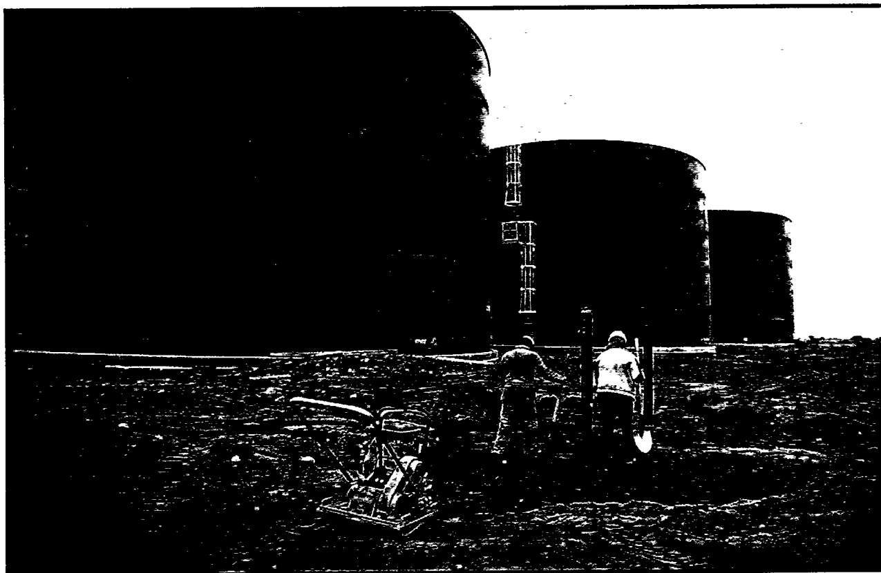
A wastewater-treatment facility under construction at Hanford to treat low-level condensate from an evaporation process that reduces the volumes of high-level waste. Each of these three tanks has a capacity of 670,000 gallons. Because of the use of this facility, the Department has ceased discharges of contaminated waste water to the soil for the first time in more than 40 years. Hanford Site, Washington. December 19, 1993.
