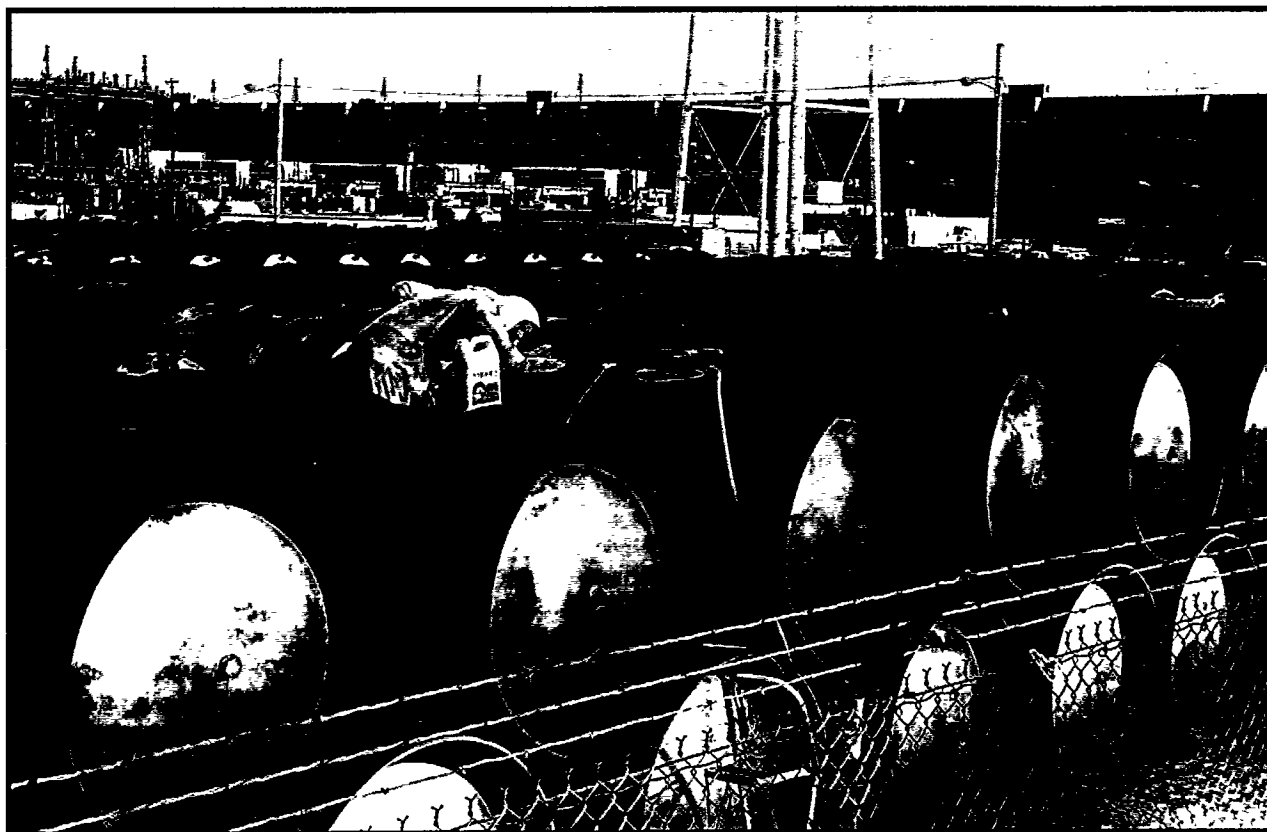
Uranium hexafluoride cylinders are stored near the K-25 Gaseous Diffusion Plant. Each cylinder contains 10 to 14 tons of depleted uranium hexafluoride. The K-25 plant stores about 5,000 of these cylinders, some of them 40 years old. Here, a worker is using ultrasound to evaluate the effects of external corrosion on a steel cylinder. Cylinders closest to the ground can experience accelerated corrosion. K-1066K Cylinder Storage Yard, K-25 Site, Oak Ridge, Tennessee. January 9, 1994.
