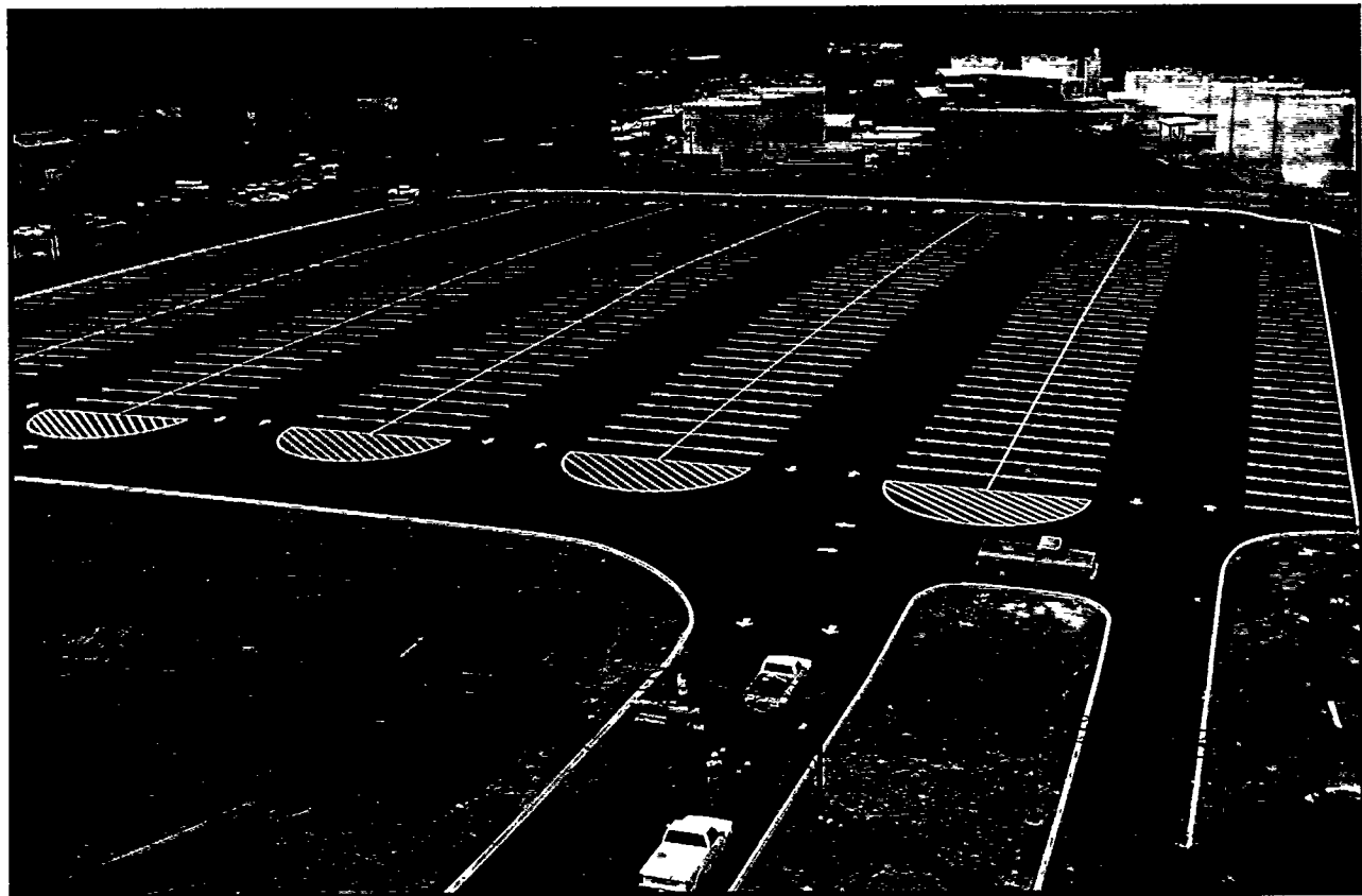
AFTER – A parking lot is now located where the four ponds shown above once stood. The liquids in these ponds were treated to remove contaminants beginning in 1985; the ponds were then drained and capped with asphalt. The project was completed in 1990. Oak Ridge, Tennessee.
