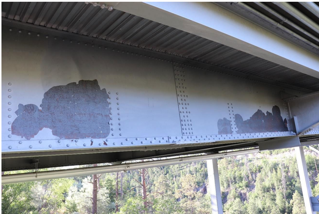
LANL 24: (b) West spandrel girder (typical): paint peeling on web and minor corrosion
