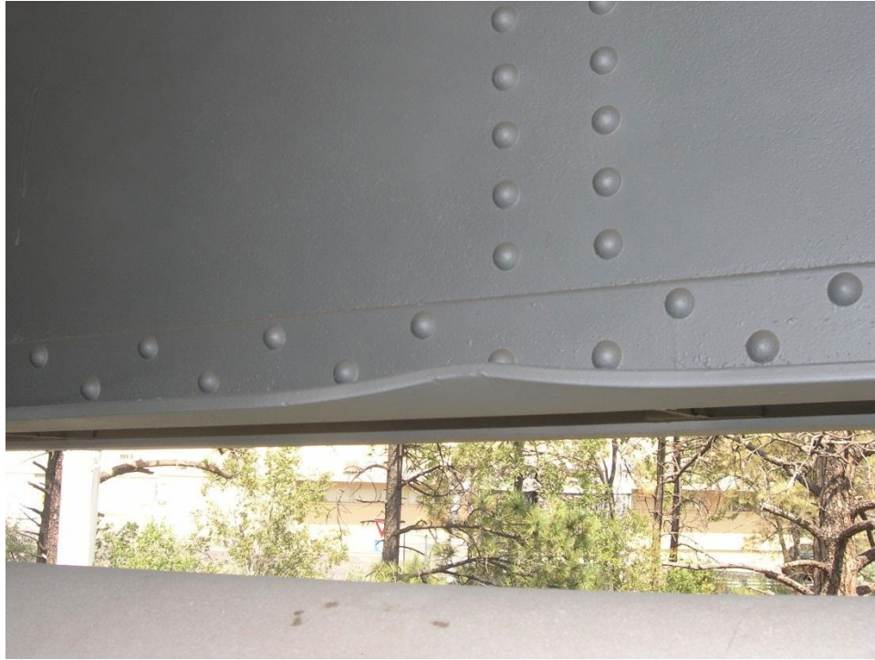
(a) East spandrel girder: impact damage to bottom flange angle (2012)
