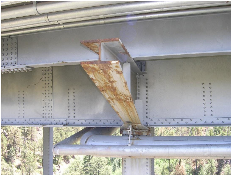
LANL 26: (b) West outrigger beam (typical): paint failure / heavy corrosion of beam and corrosion / pack rust / distortion at bottom channel connection to column (2013)
