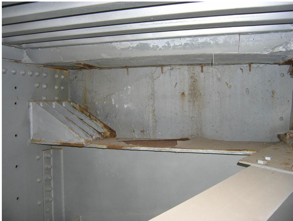
LANL 18B: Paint failure / corrosion on west outrigger TF at south abutment (2014).
