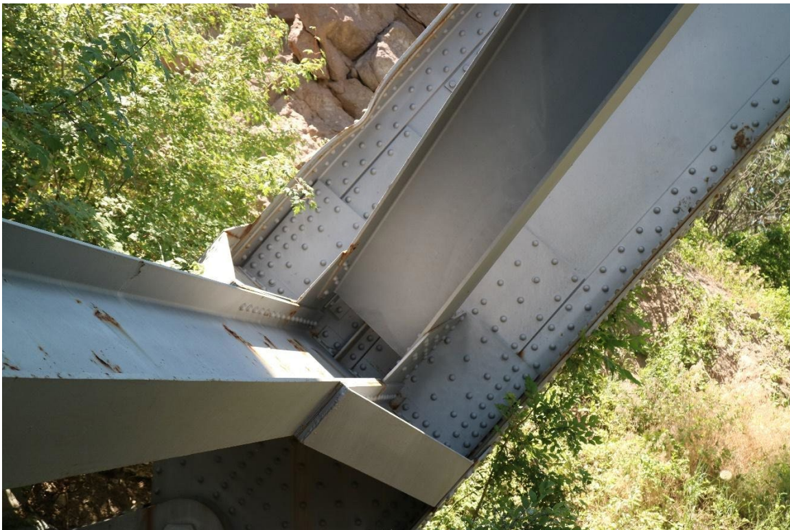
LANL 25: (b) Arch rib: impact damage to top plate (2018)
