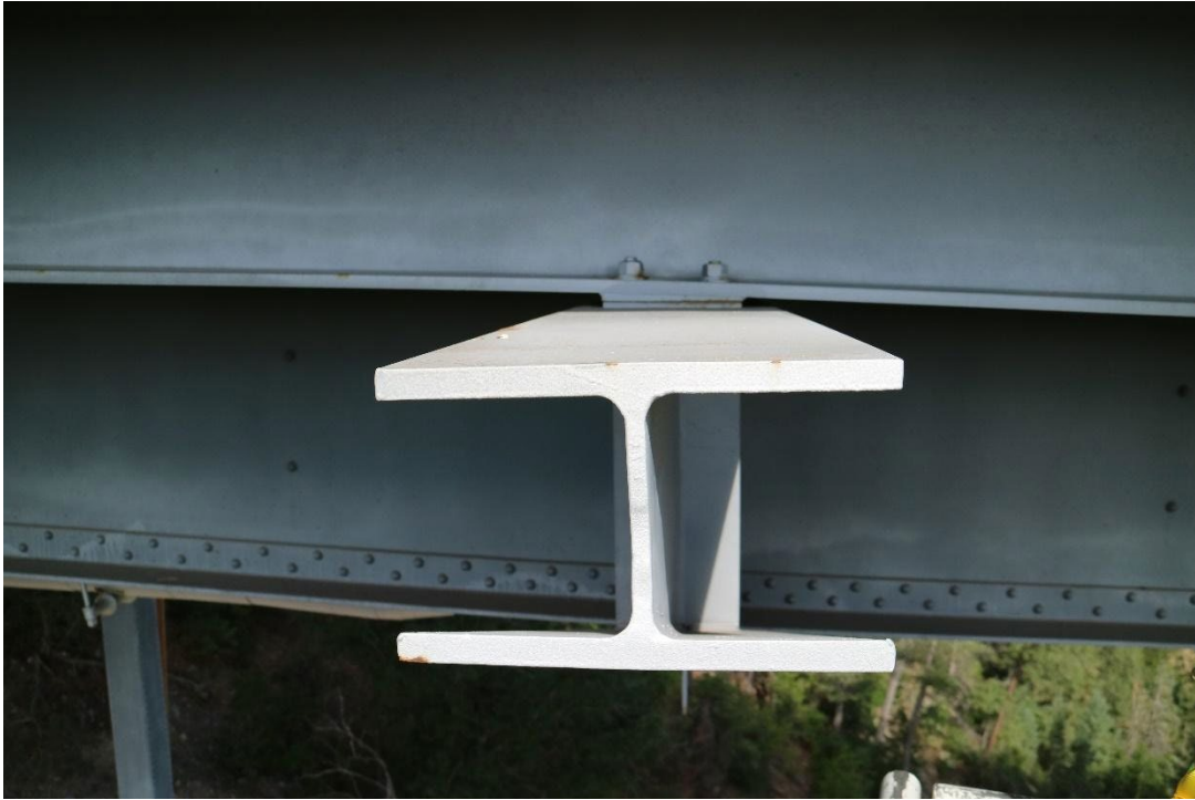
(a) Distortion (typical) of outriggers (2016)
