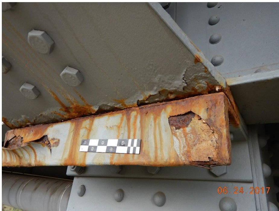
LANL 29: (b) East arch, column 8, knee brace at floor beam 15, outside face, typical corrosion
