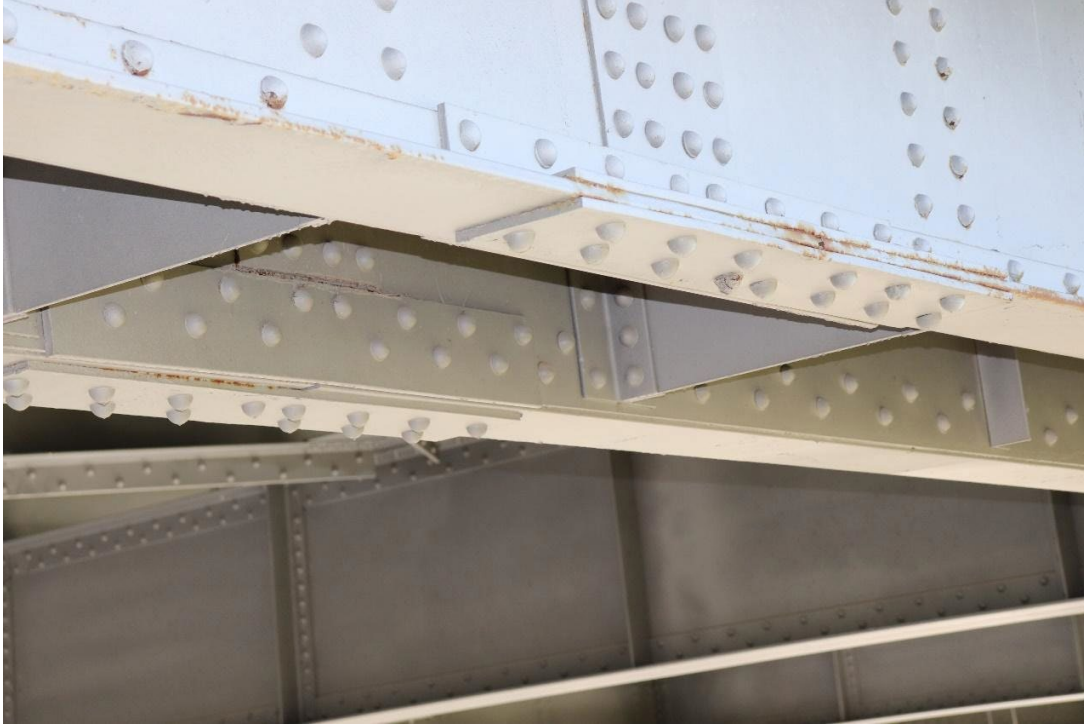
LANL 18A: Corrosion / pack rust on BF splice connection at west spandrel girder (2014).
