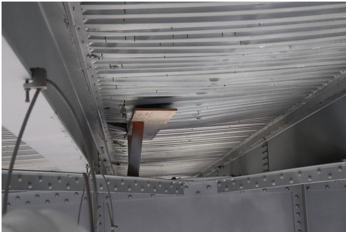
LANL 27: (b) Stay-in-place forms: note haphazard support by timber shoring
