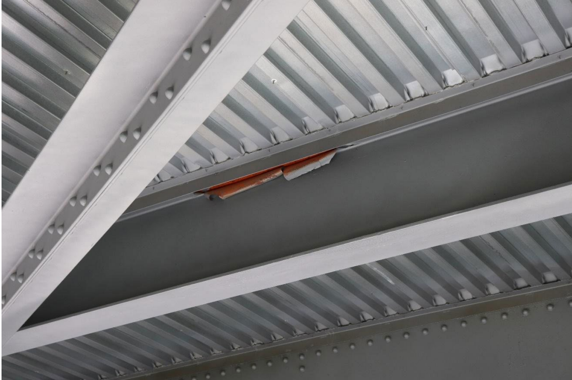
(a) Stringer: note leaching, paint failure, and corrosion at top flange
