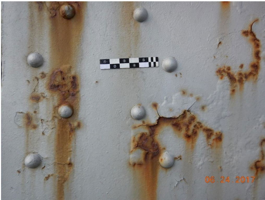
LANL 28: (b) East Arch, typical paint peeling/cracking and surface corrosion on top flange
