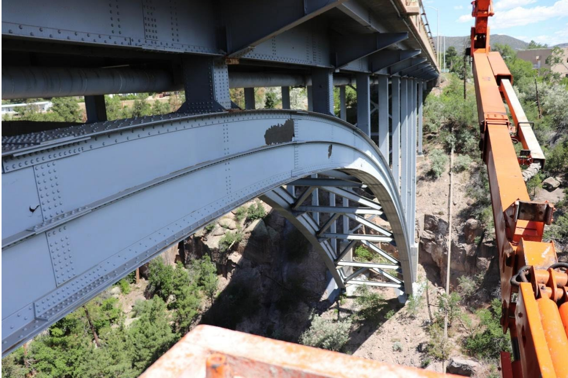
(a) East arch rib (typical): minor paint peeling on web
