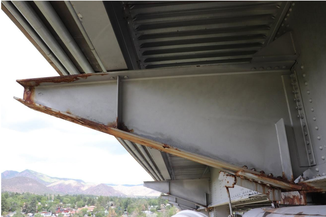
(a) West outrigger beam (typical): paint failure / moderate corrosion of beam and corrosion / pack rust / distortion at bottom channel connection to column
