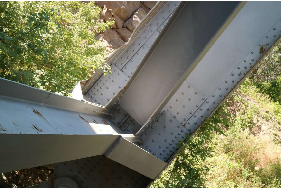
Arch rib: impact damage to top plate (IMG_3771 [2018])
