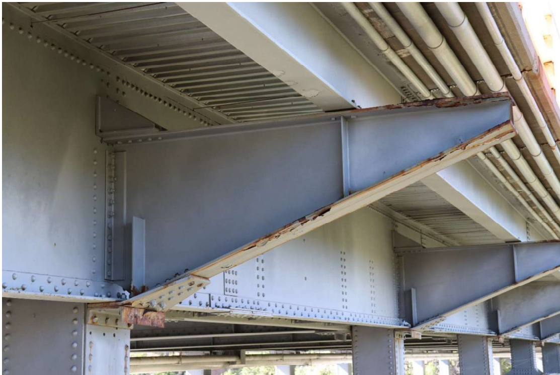
West outrigger beam (typical): paint failure / moderate corrosion of beam and corrosion / pack rust / distortion at bottom channel connection to column (IMG_0262)
