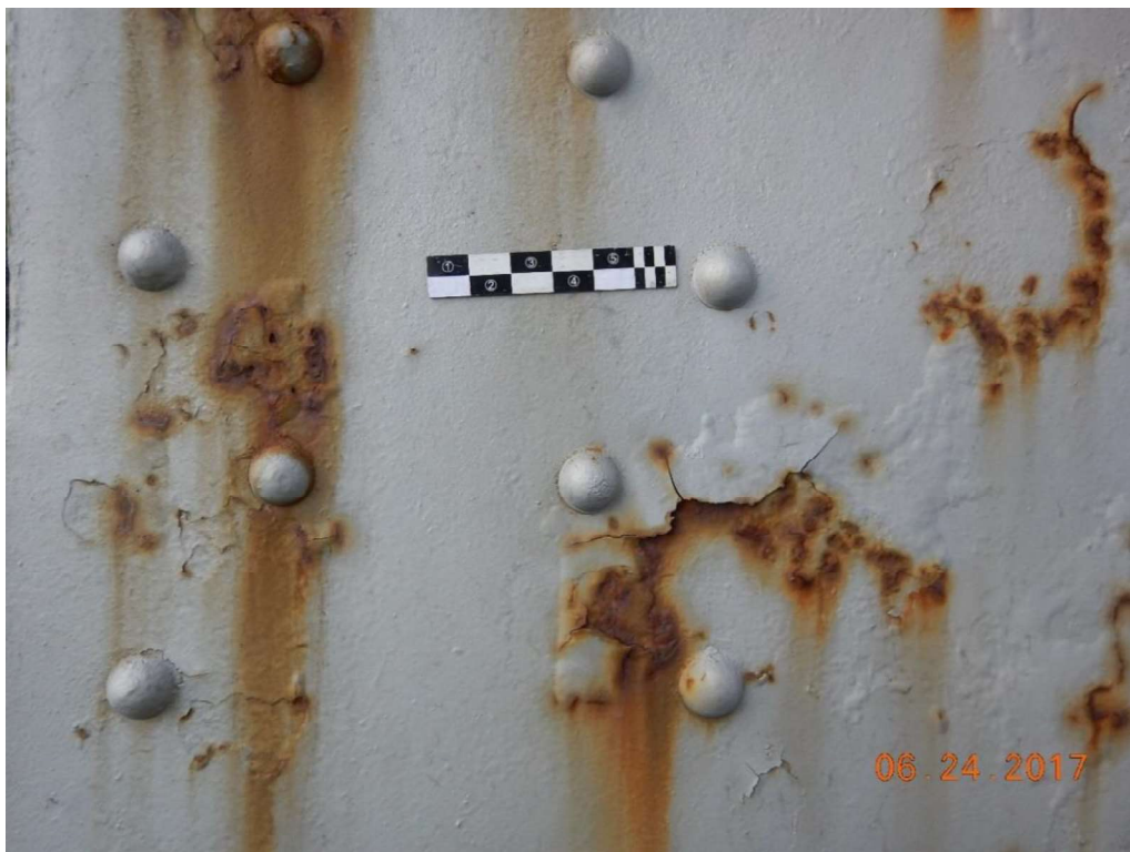
East Arch, typical paint peeling/cracking and surface corrosion on top flange
