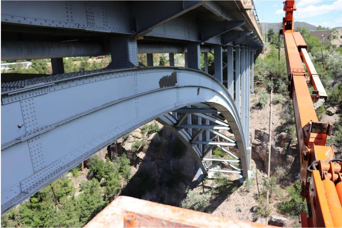
East arch rib (typical): minor paint peeling on web (IMG_0180)
