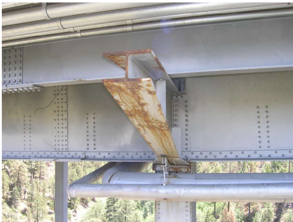
West outrigger beam (typical): paint failure / heavy corrosion of beam and corrosion / pack rust / distortion at bottom channel connection to column (2013)
