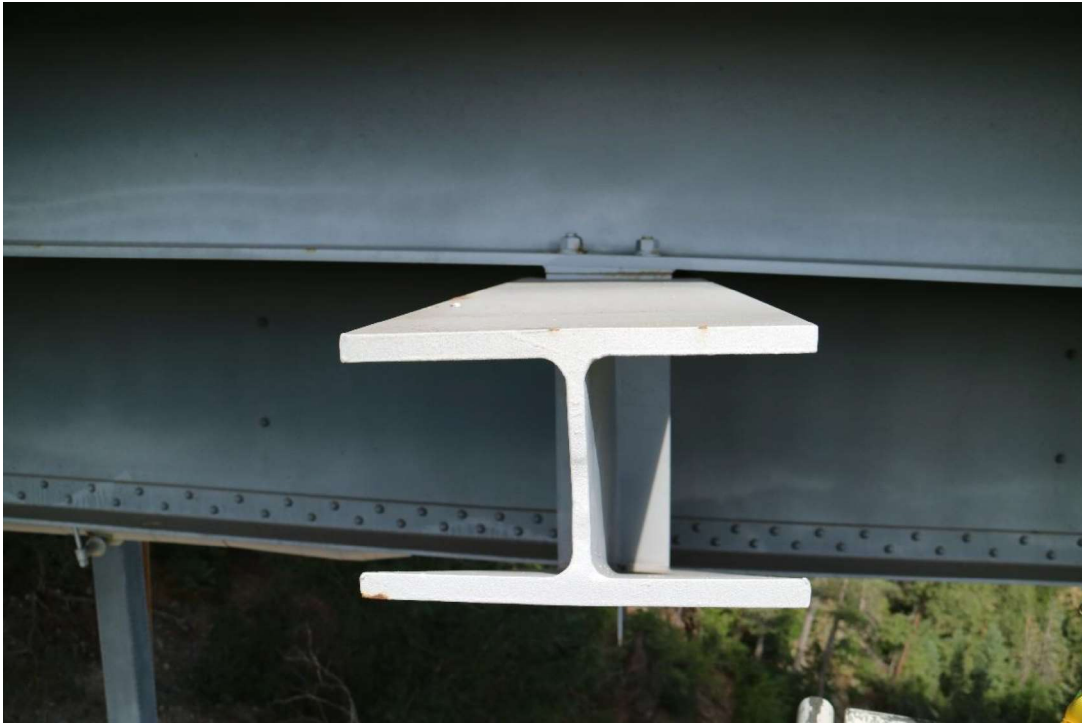
Distortion (typical) of outriggers (2016)
