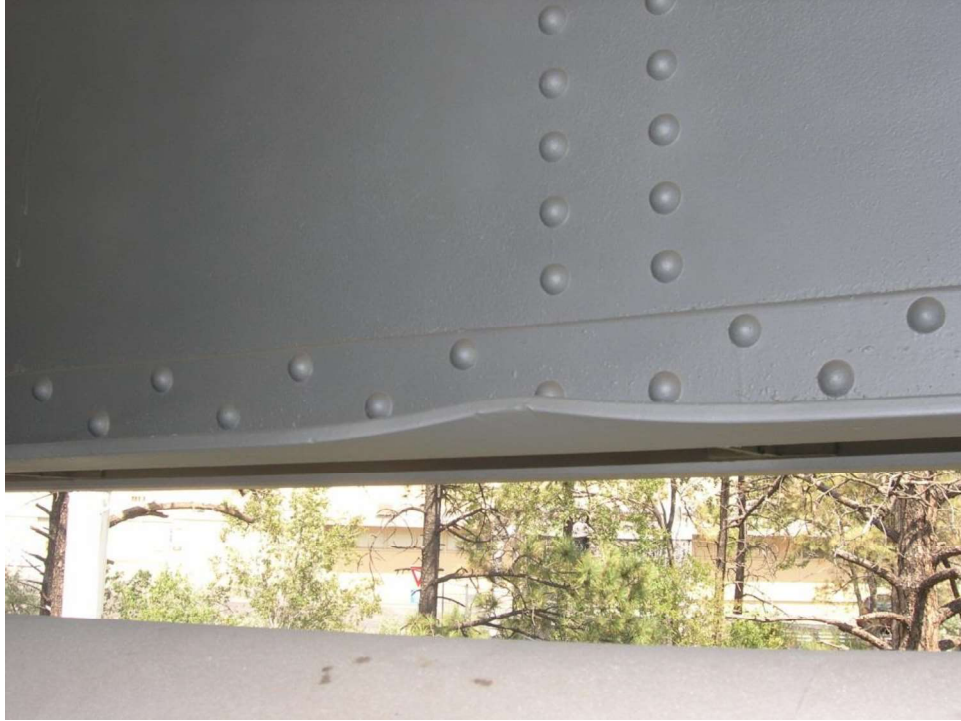
East spandrel girder: impact damage to bottom flange angle (2012)
