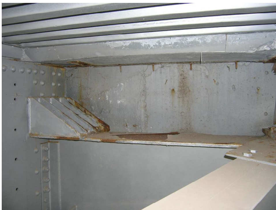
Paint failure and corrosion on west outrigger top flange at south abutment (2014).
