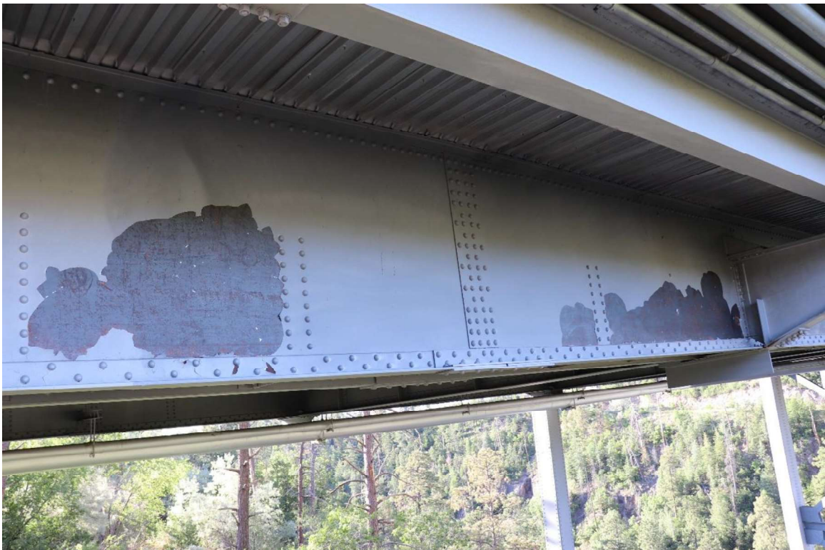
West spandrel girder (typical): paint peeling on web and minor corrosion (IMG_0215)
