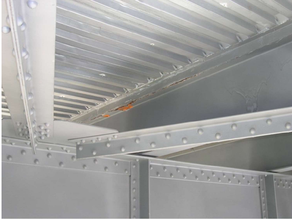
Stringer: note leaching, paint failure, and corrosion at top flange (2012)
