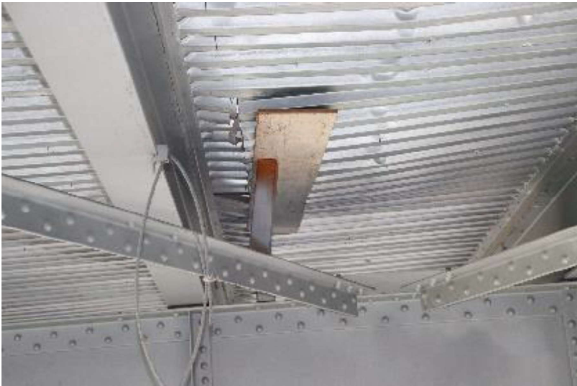
Stay-in-place forms: note haphazard support by timber shoring (IMG_0173)
