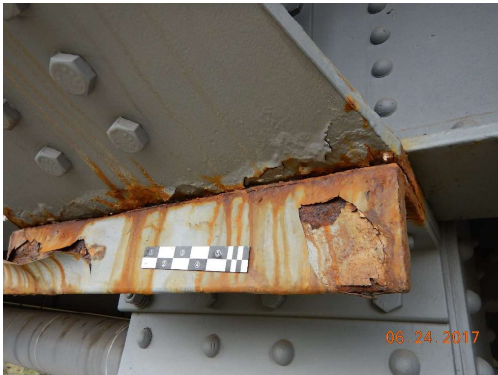
East arch, column 8, knee brace at floorbeam 15, outside face, typical corrosion
