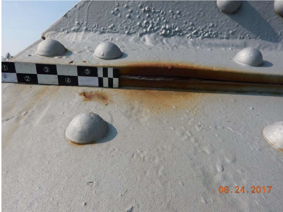
East arch, column 14, 1/16" pack rust at base
