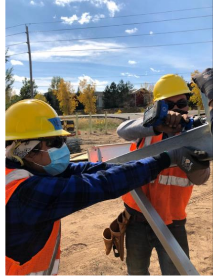
Figure 3. Trainees on-site in BP2.
