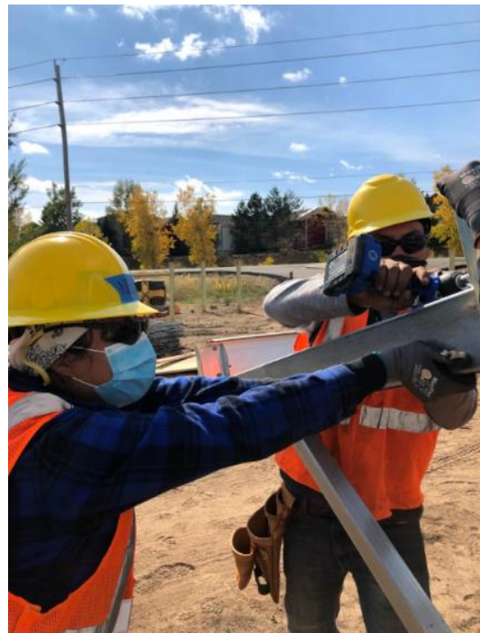
Figure 8. Trainees working during BP2.
