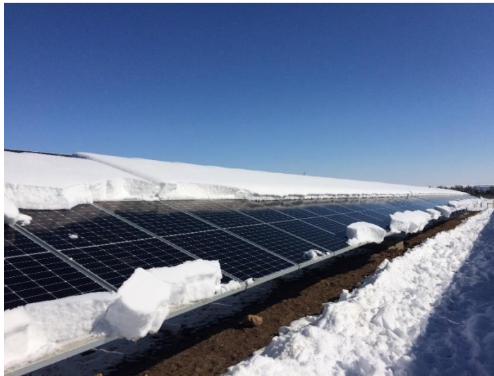
Figure 5. Weather intervenes at the Boulder, Colorado, installation in BP1.
