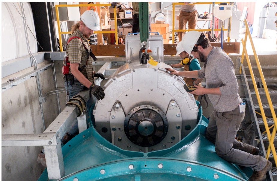
Figure 13: installing a direct drive PMG into Natel's prototype axial flow D190 turbine.
