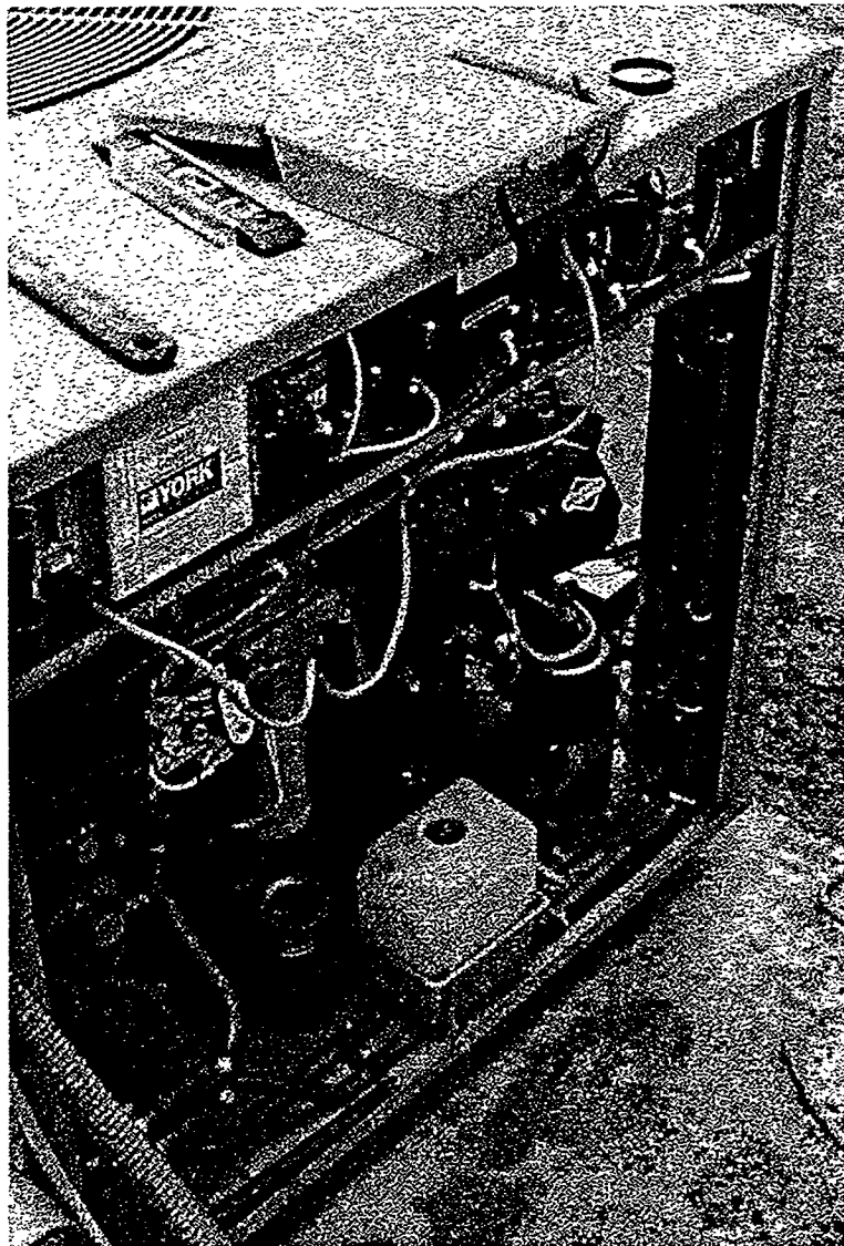
Figure 3. Triathlon GHP Outdoor Unit With Back Panel Removed
