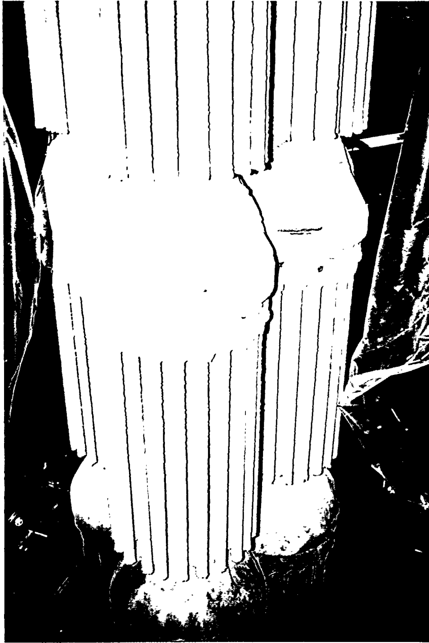
Figure 4.3.4 - Photograph of Filter Internals Following Test Run 4
