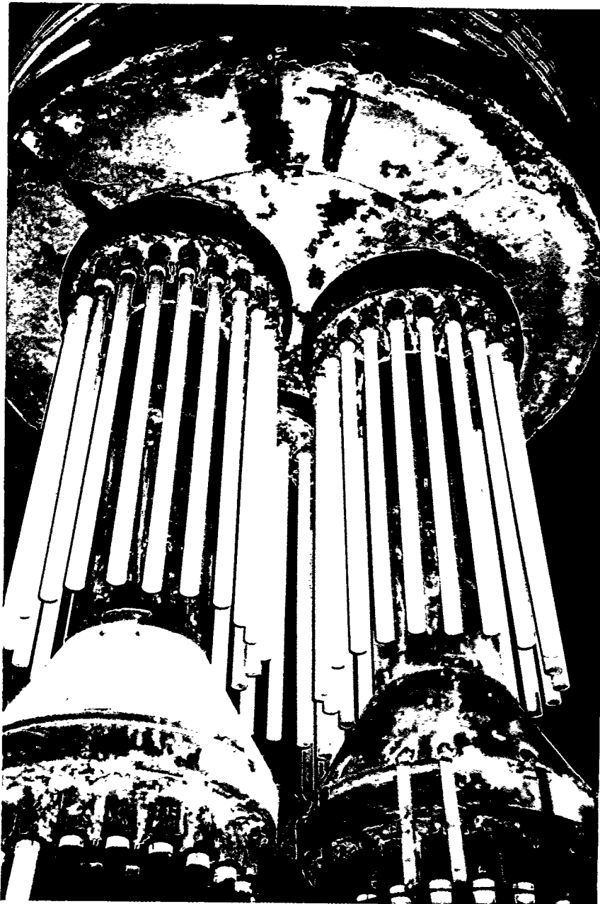
Figure 4.5.19 - Photograph of Filter Internals Before Test Period IV
