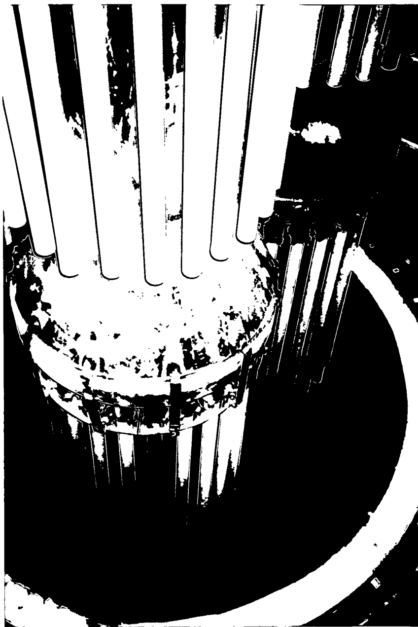
Figure 4.5.24 - Photograph of Filter Internals Before Test Period IV
