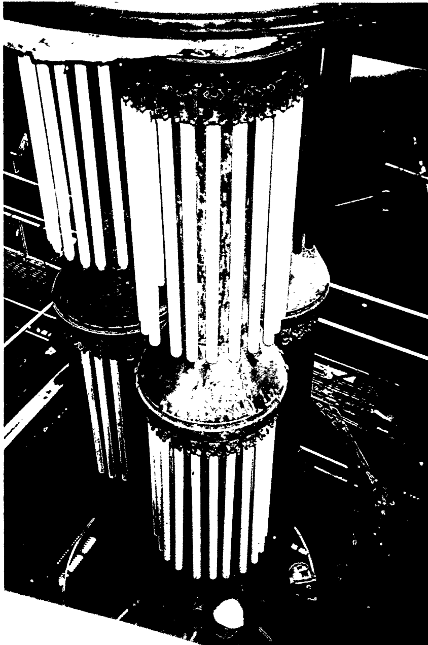
Figure 4.6.20 - Photograph of Filter Internals Before Test Period V
