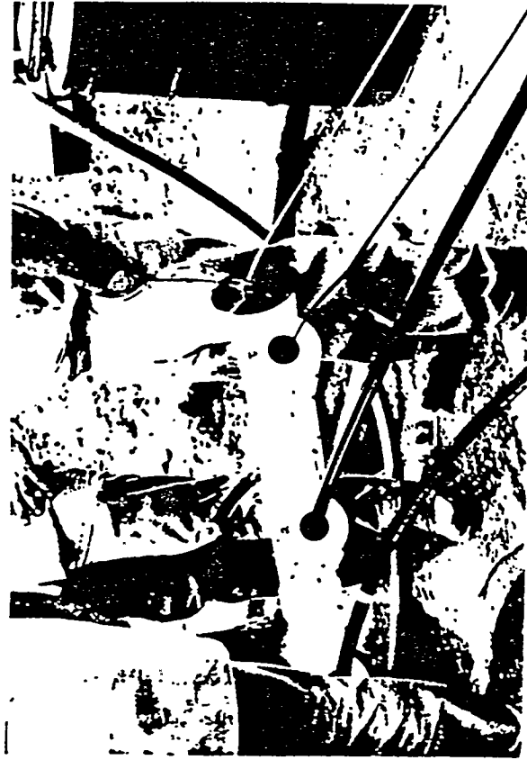
c) End View of Casing Showing Service Lines, Pull-In Cable and Super Vacuum
