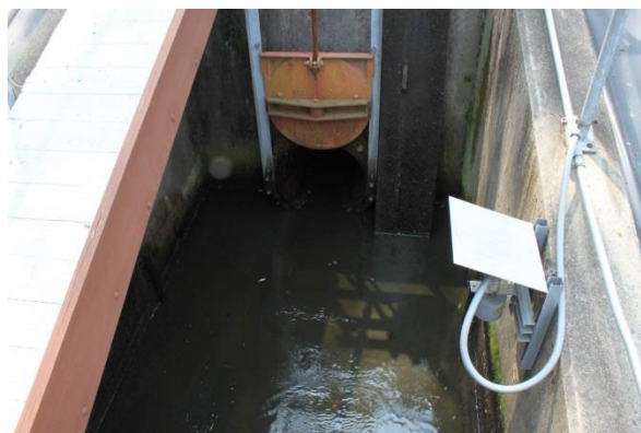
Exhibit 4-4. Flow Sensor and Discharge Valve
