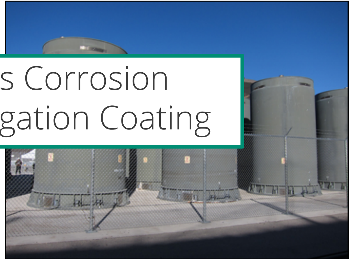
Vertical canisters in concrete overpacks Bryan & Enos, SAND2014-203470
