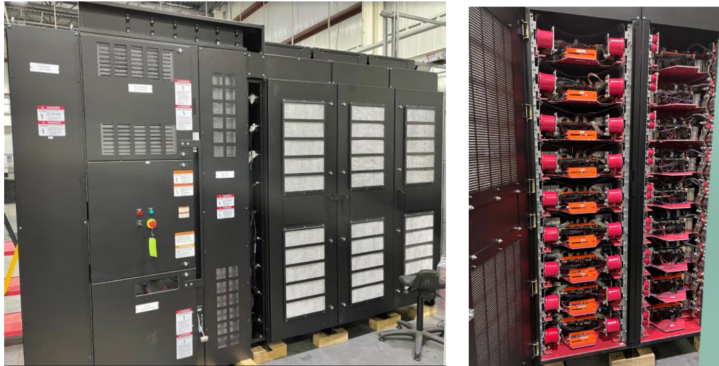
Fig.8.4.1 1 MVA M4 Inverter system. Right hand side picture shows the modular converters.
