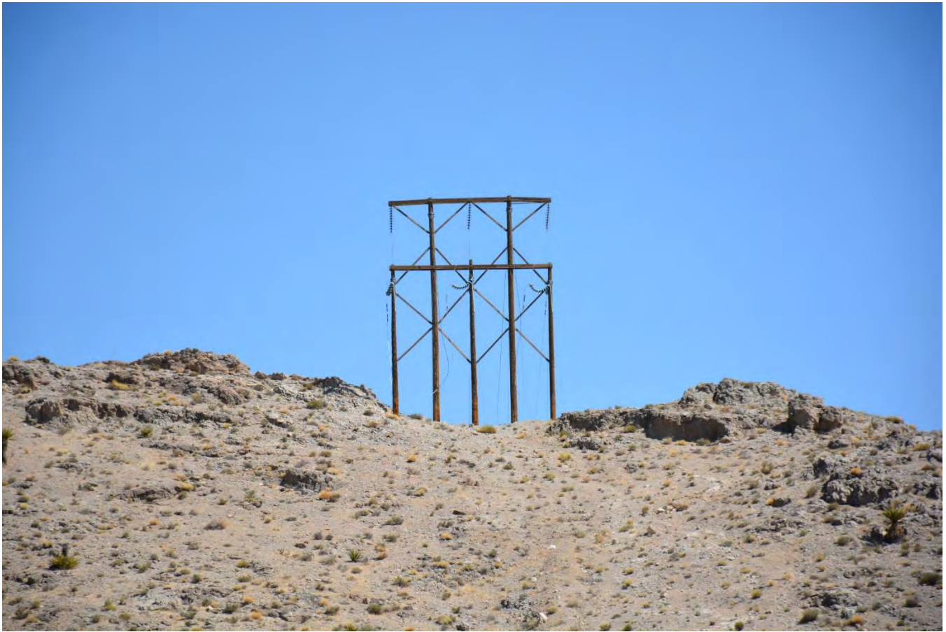
Figure 12-7. Historic 138-kilovolt high tension suspension structure on hill crest at Checkpoint Pass, facing north-northwest (DRI 2022)
