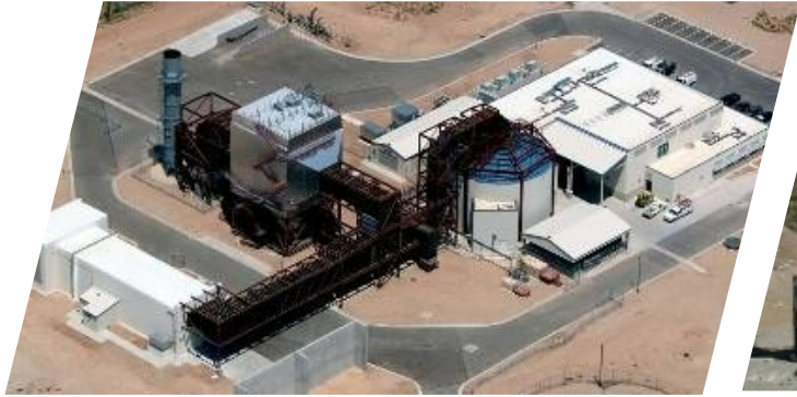
THERMAL TEST COMPLEX
