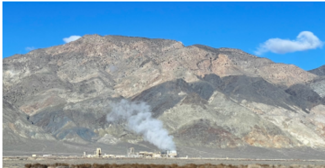
Dixie Valley Geothermal Plant
