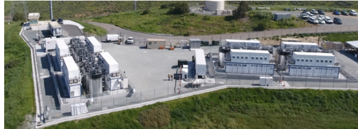
Sumitomo 2MW/8MWh vanadium Redox Flow Battery system in San Diego, CA
