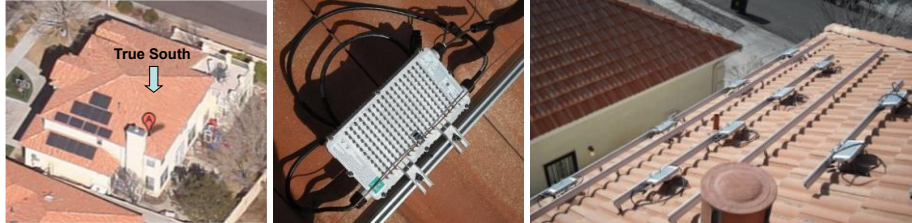
Figure 1. 3 kW photovoltaic installation in Albuquerque, NM, using Enphase’s first-generation microinverters.
