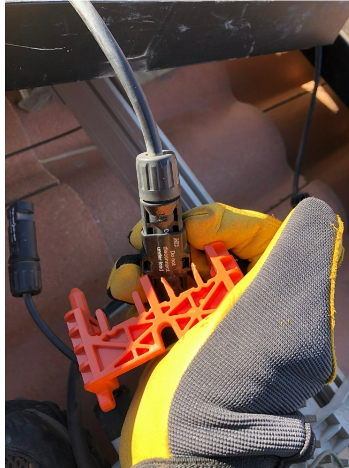
Tool did not fit in slots for negative coupler
