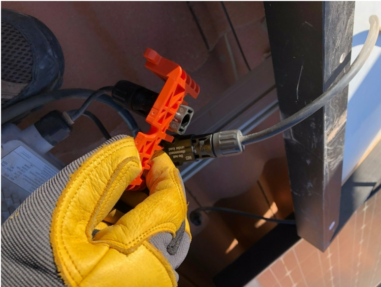
Positive coupler came apart easily with special tool
