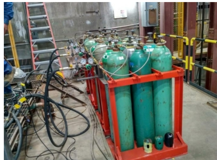
Pressurized gas supply (18 bottles)
