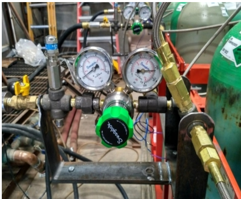
Manifold regulator for gas supply
