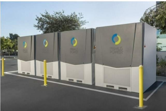
Primus Power modular Zn-Br, each unit is 25kW/125kWh
