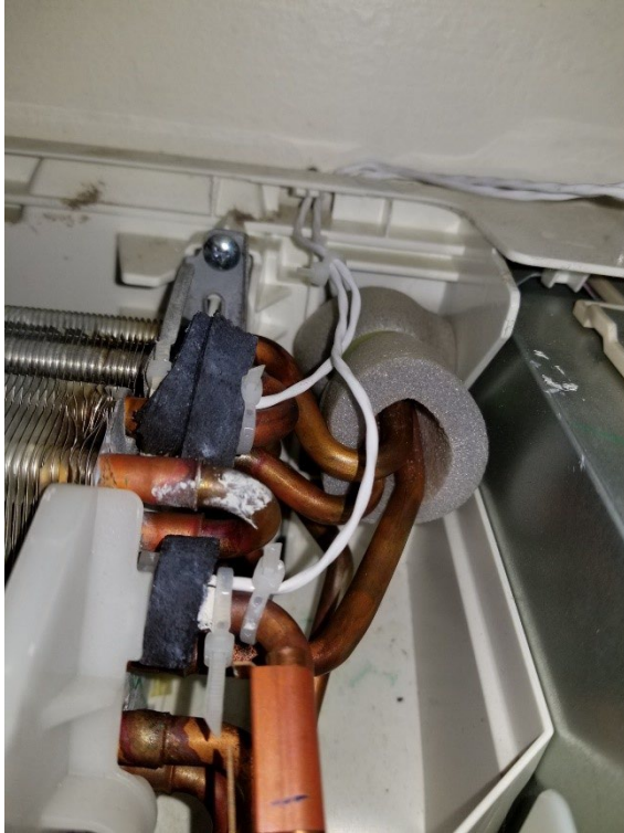
Figure 63: Original liquid line thermistor that was installed incorrectly in February 2021
