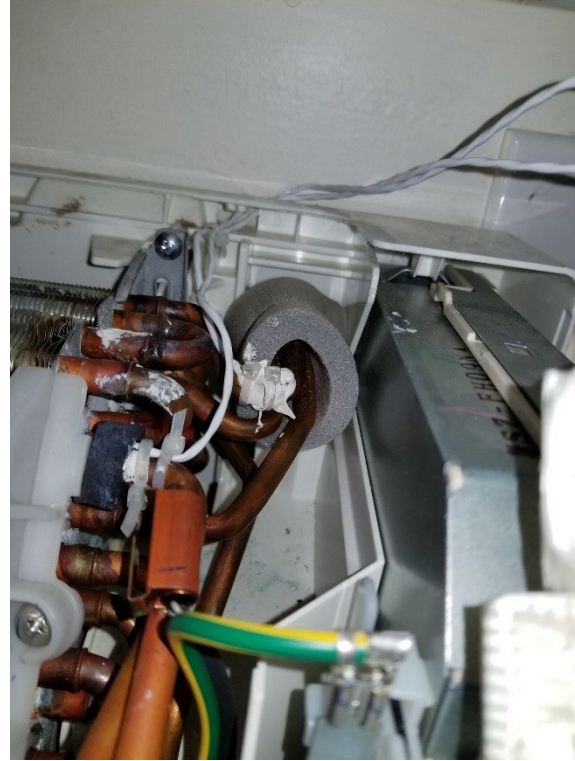
Figure 64: Liquid line thermistor moved to correct position on October 28 th , 2021
