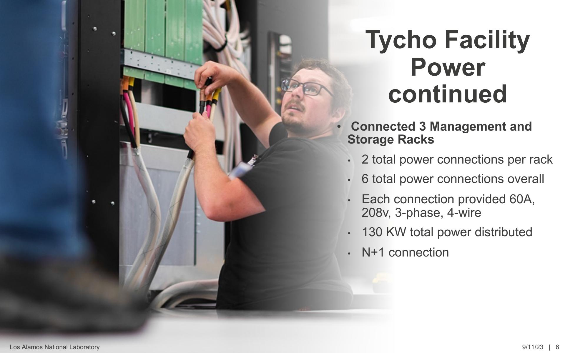
A photograph of a man with a beard and glasses, wearing a black t-shirt, working on a server rack in a data center. He is holding a power cord and connecting it to a rack-mounted power distribution unit. The rack is filled with green server modules and various cables. The background is a blurred view of the data center's interior.
