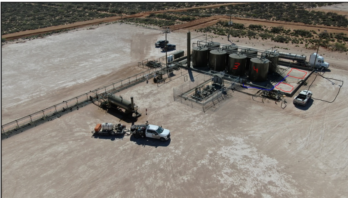
Figure 3. Tanks #3 & #4 contained the produced water that was treated. Treated water was pumped back into tank #4.
