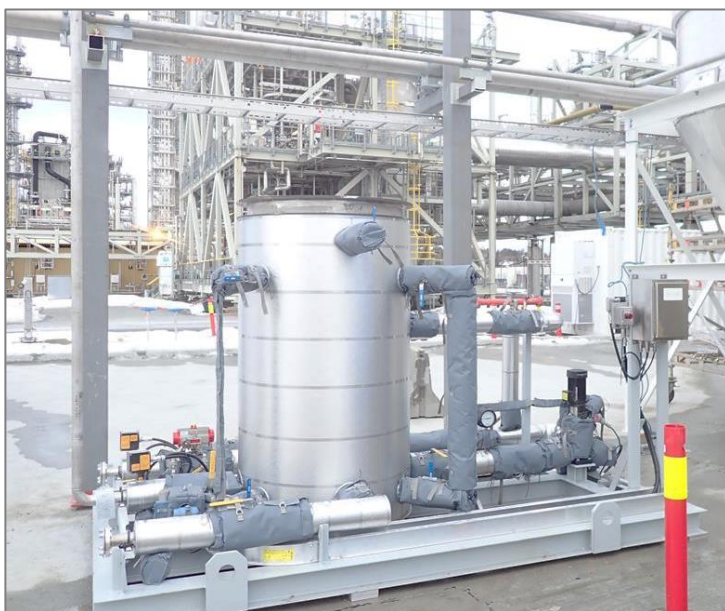
Figure 25. A photo of the wastewater skid at the TCM third site during initial installation activities in January 2021.
