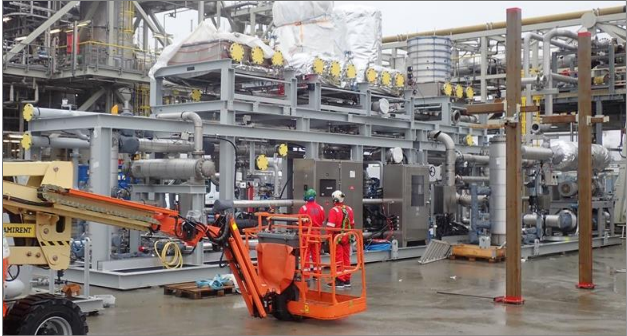
Figure 35. The main skids of the MTR test system ready for removal from the TCM third site during decommissioning activities.
